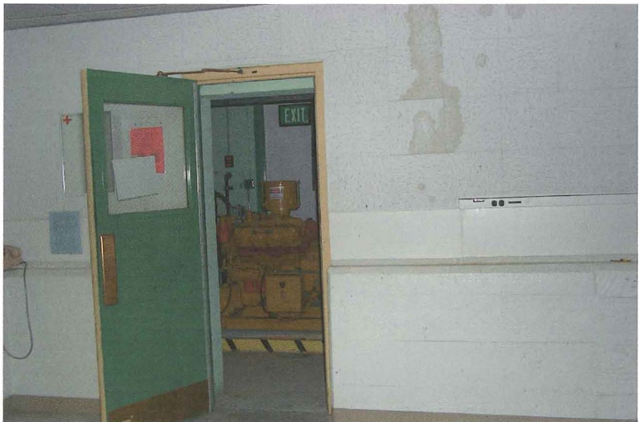
TA-2-1, Rooms 116 & 116A
