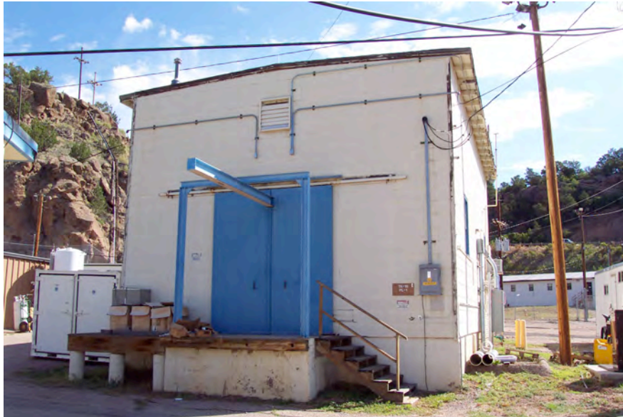
Figure 15.9. Building 18-1, site of a fatal criticality accident.
