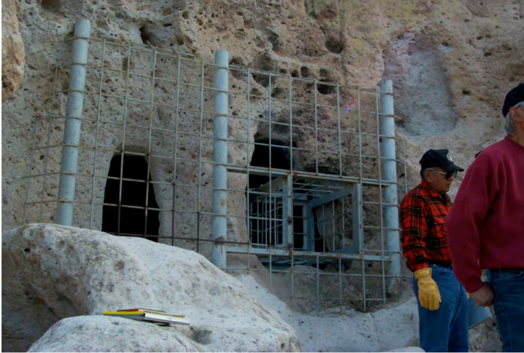
Figure 15.15. Steel grate in front of Mortandad Cave Kiva.
