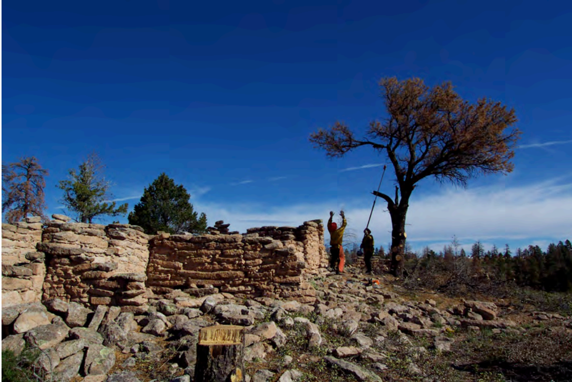
Figure 20.2. Overhanging branches are removed from a snag at Nake'muu to minimize chance of damage to standing walls.
