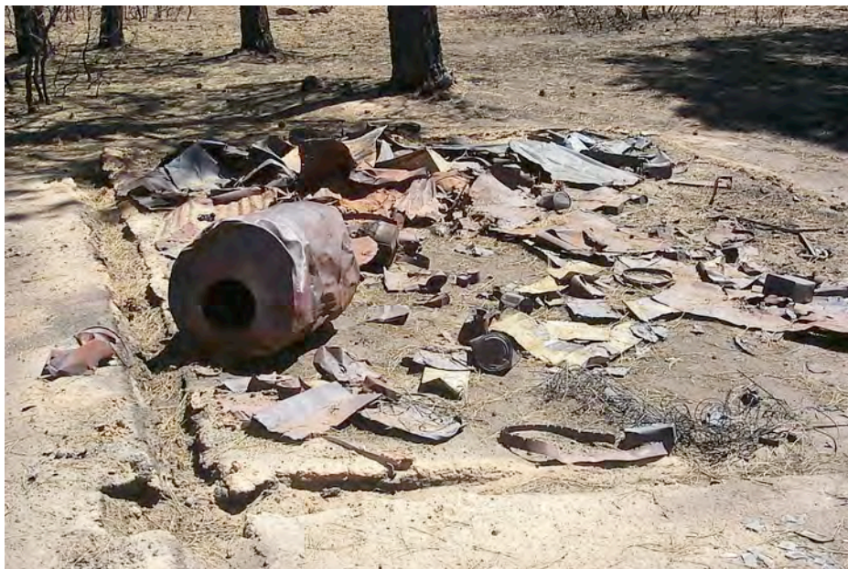
Figure 5.4b. Homestead depicted in Figure 5.4a after the Cerro Grande fire.
