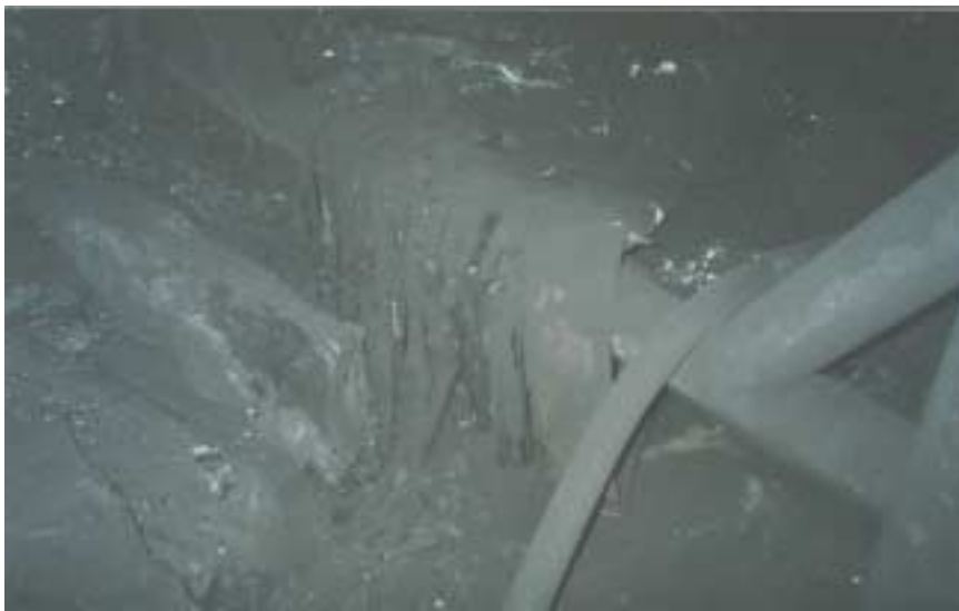
Figure 31: Located in the #3 entry along the inby ribline of the last open crosscut between spad #13352 and spad #13353. Picture of melted resin cartridges on the supply sled.
