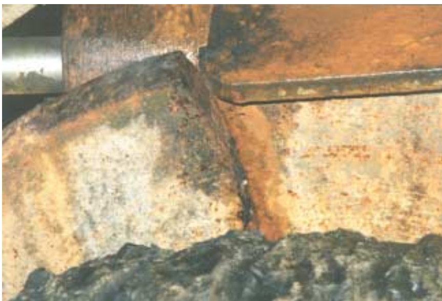
Figure 4: Crack in frame on the bucket end of scoop (inby side).
