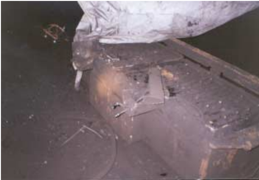
Figure 9: Scoop battery located in the last open crosscut between #2 entry (spad #13352) and #1 entry (spad #13349). This battery was found upside down during recovery operations.
