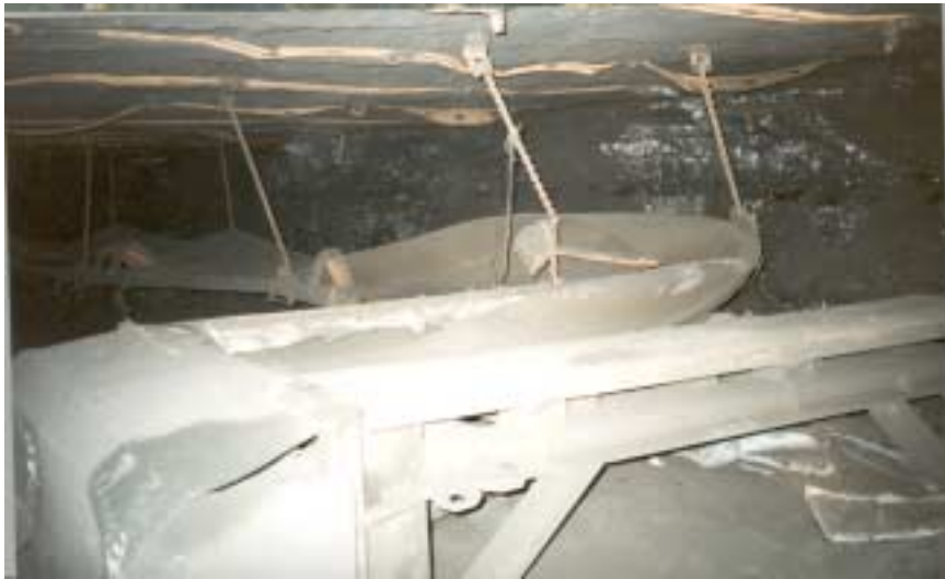
Figure 5: Conveyor belt tail-piece looking outby from spad #13346.
