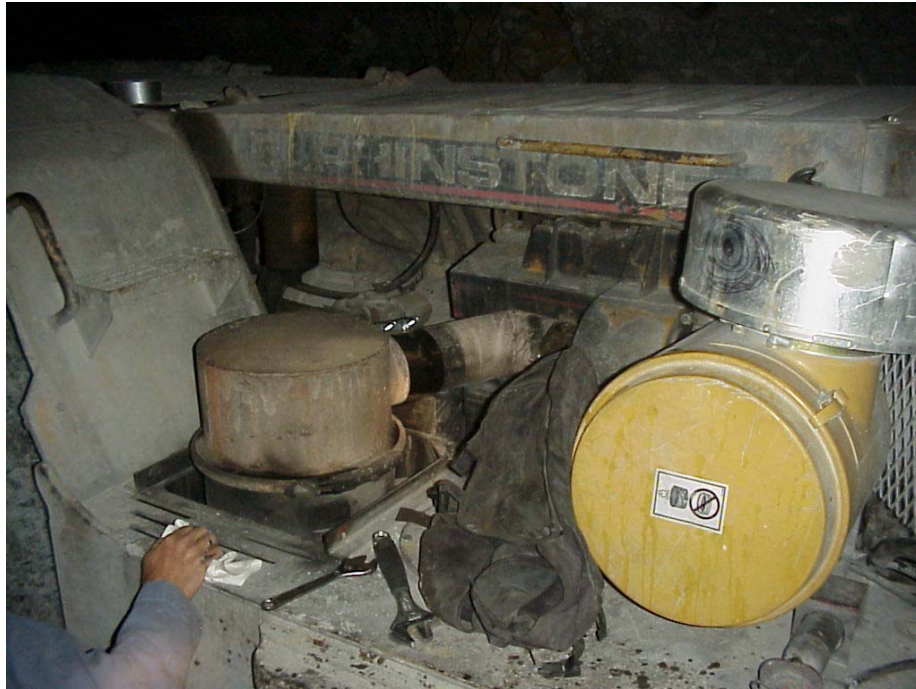
Figure 2. Passive DPF Mounted on LHD at Deep Post Mine.
