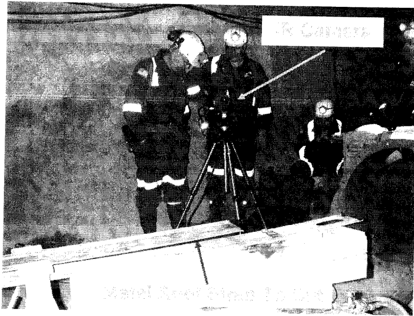
FIGURE 7. INFRARED CAMERA POSITIONED TO VIEW METAL ROOF STRIPS TO BE CUT
