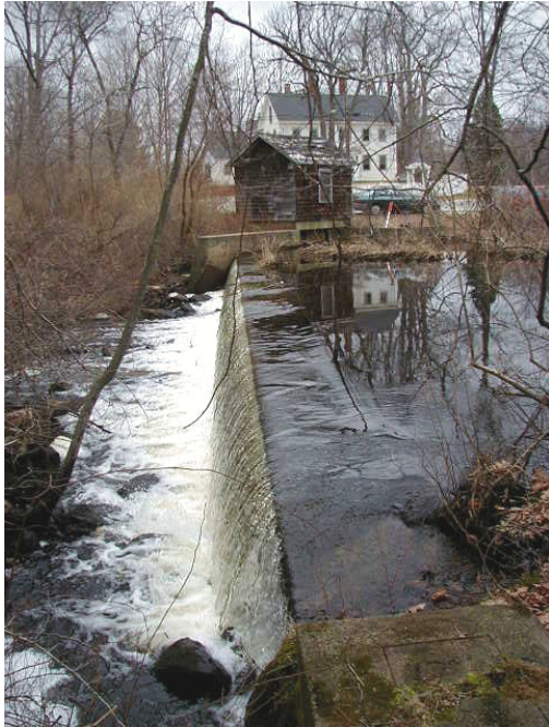
Main Street Dam on the Parker River.
