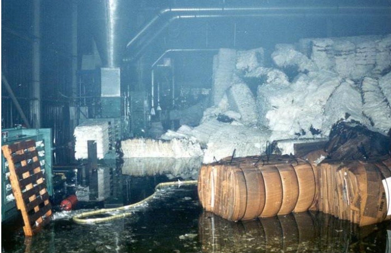
Photo 2. Paper Bales Which Caught Fire; Area Where Fire Fighters Entered Through the South-End Door With Hoselines.
