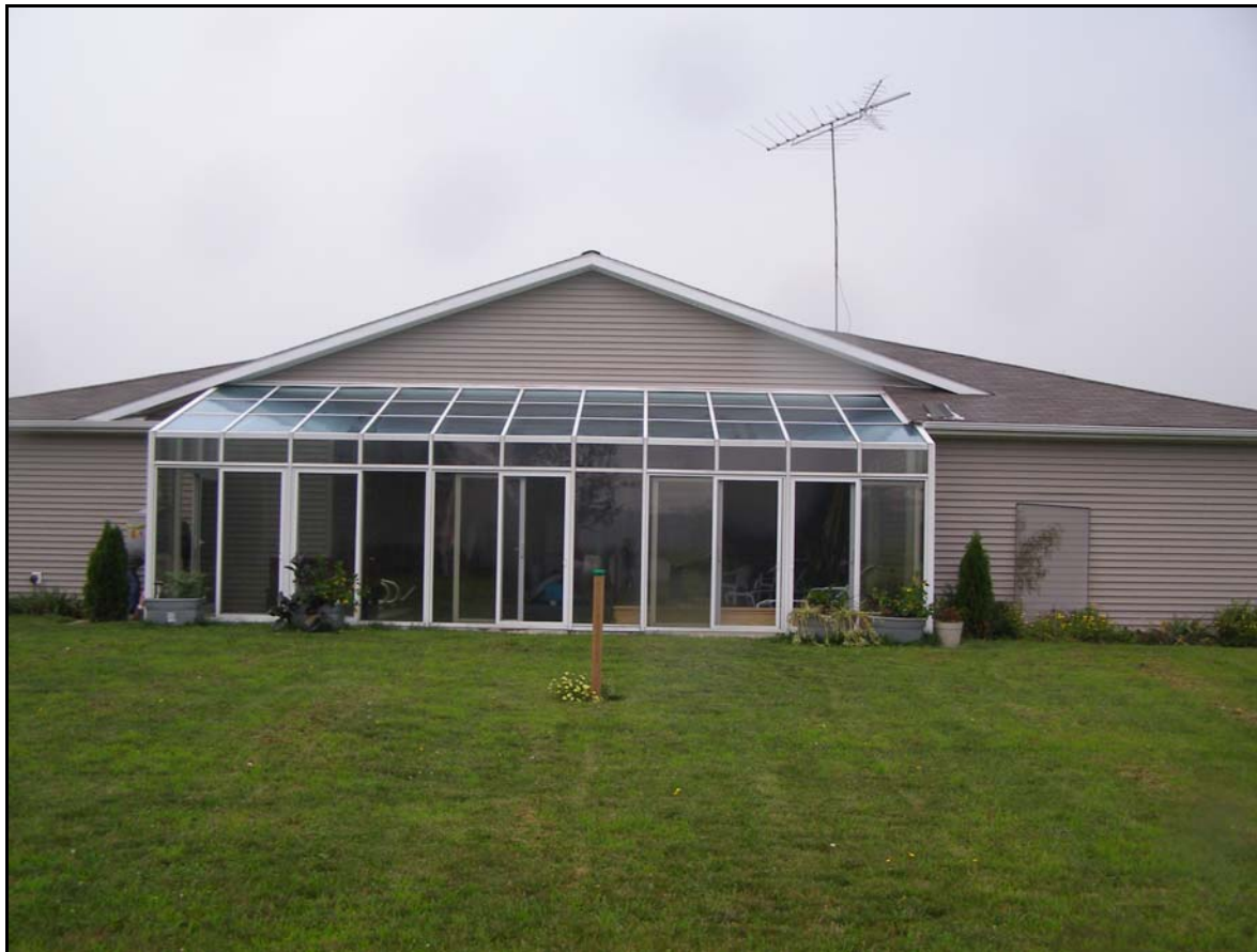
Photo 1: Side-C of the structure. Photo courtesy of the fire department.
