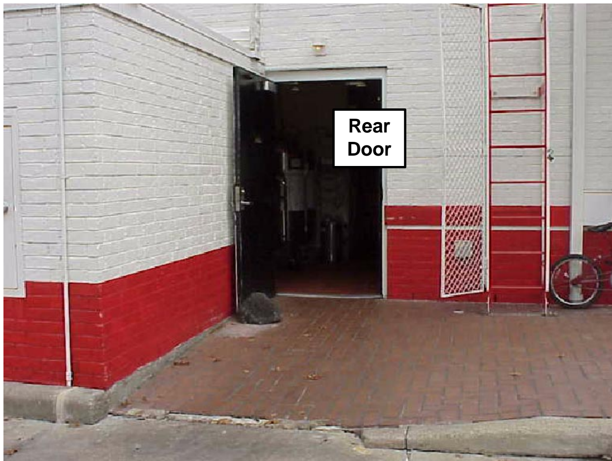
Photo 10. Rear Door Used by Fire Fighters to Gain Access During Search for Victims Note: Photo was taken of a restaurant similar to the one involved in this incident.
