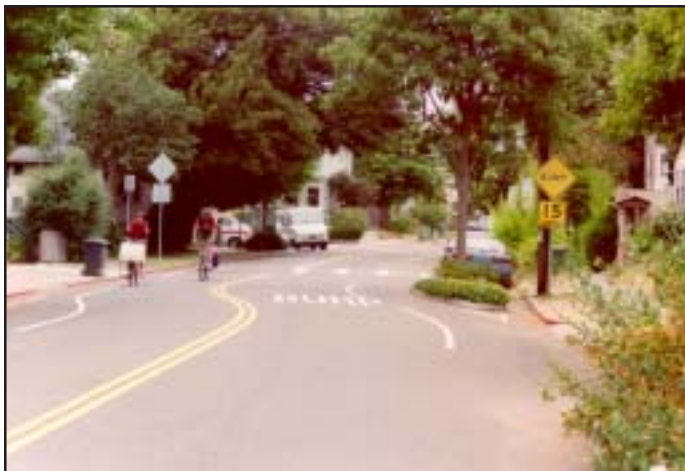
Figure 4.3: This chicane of staggered landscaping on both sides of the street creates curves that encourage drivers to slow down.
