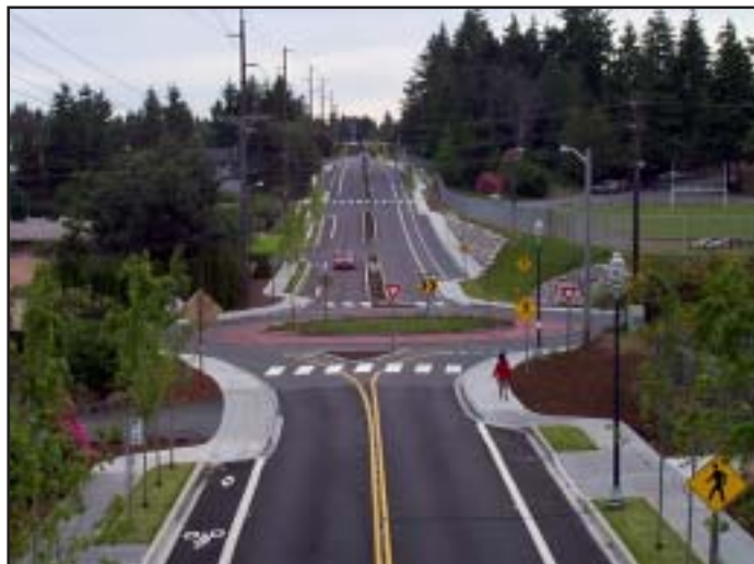
Figure 4.1: The addition of bicycle lanes and sidewalks create space for pedestrians while medians and landscaping narrow the street width and slow traffic.
