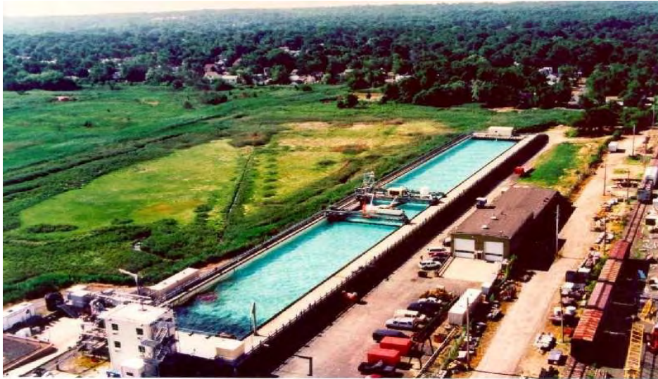
Figure 21: Ohmsett Facility in New Jersey
