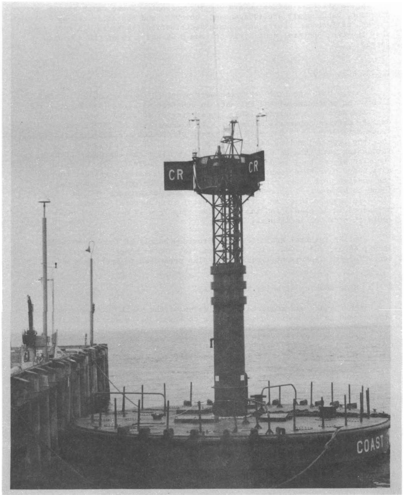
Figure 4. NOAA data buoy 46010 at dockside in Astoria, Oregon.
