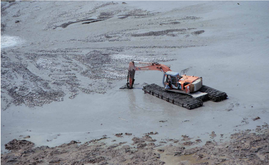
▲ Figure 4. Marsh buggy inside containment area moving sediment away from discharge pipe. (Photo courtesy of Dr. Erik Zobrist, NOAA Habitat Restoration.)
