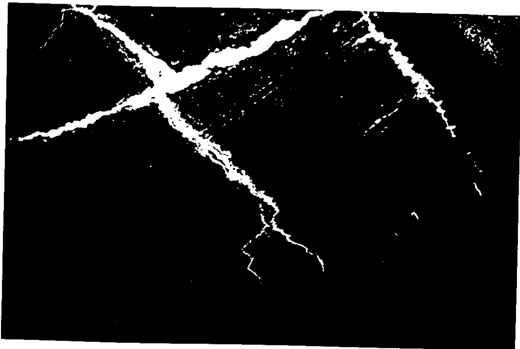
PHOTO 2. A general crack on a concrete slab
