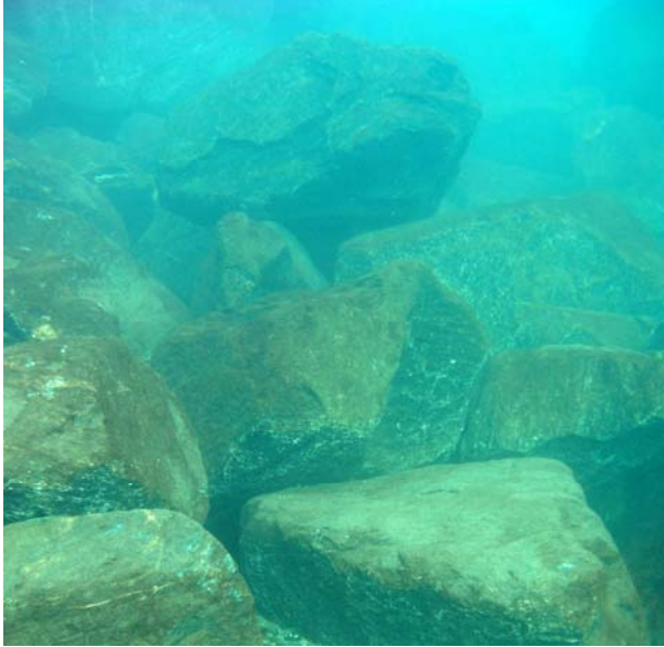
Figure 4: Boulders forming the artificial reefs in Yankee Cove, ranging in size from 0.5 to 1 meter in minimum diameter.
