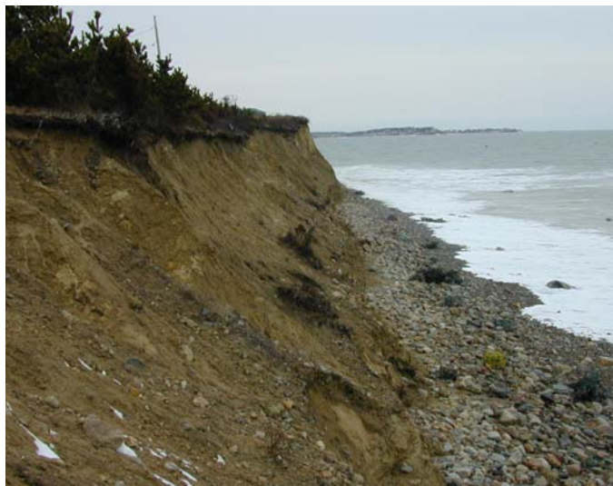
Figure D.2.9-18. Erodible bluff fronted by narrow cobble beach, Scituate, Massachusetts (Photo courtesy of R. Haney, Massachusetts Coastal Zone Management)
