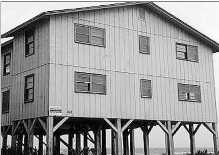
CRS communities often contain elevated buildings.
