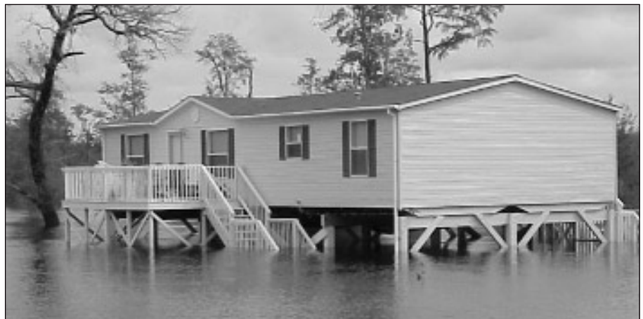
Rivers in North Carolina overflowed after Hurricane Floyd.
