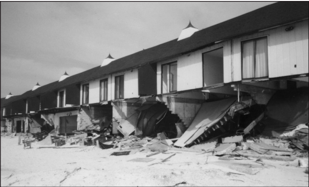
Storm surges often damage coastal condos.
