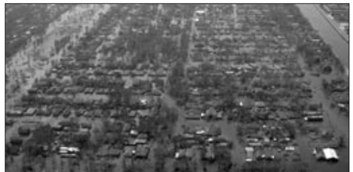
Large parts of New Orleans remained flooded for weeks after several levees failed in the wake of Hurricane Katrina. (Photo by Bob McMillan, FEMA)
