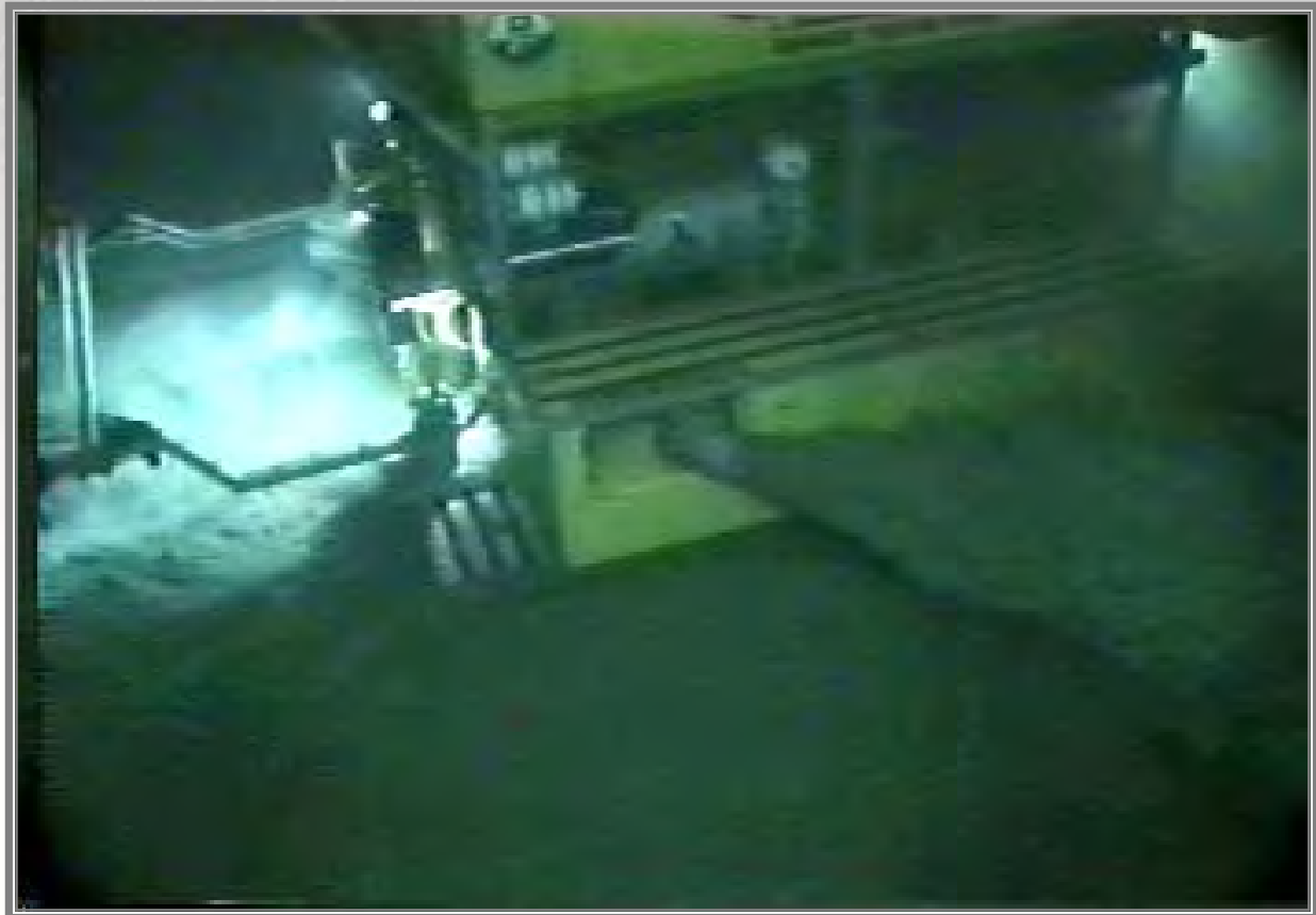
Talon / T500 Trenching on Angus
