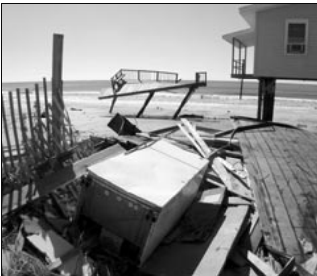
Hurricane Floyd drove a 15-foot storm surge across Oak Island, North Carolina, damaging or destroying hundreds of houses. (Photo by Dave Gatley, FEMA)
