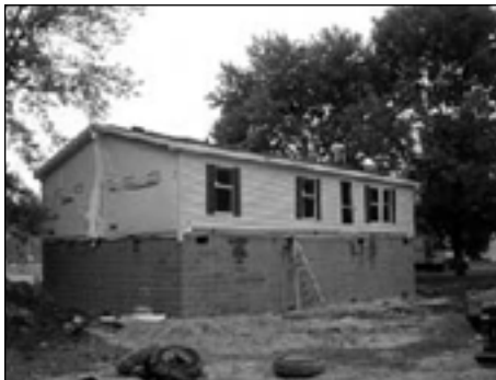
Glaze home waiting for finishing touches. (Photo by Anita Nance)
