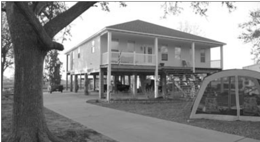
Elevated homes like this one in Pascagoula, Mississippi, which was unharmed by the Hurricane Katrina flooding that destroyed the rest of their neighborhood, stay dry well above the BFE. (Photo by Mark Wolfe, FEMA)
