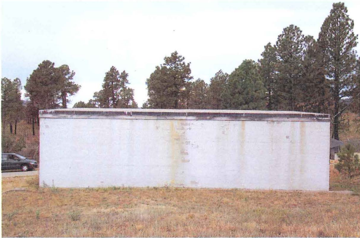
TA-37-27 Northeast Elevation
