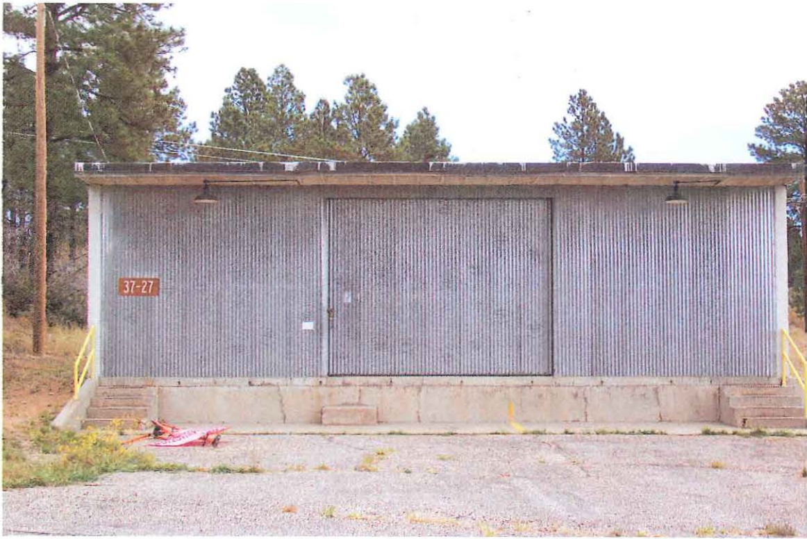
TA-37-27 Southwest Elevation
