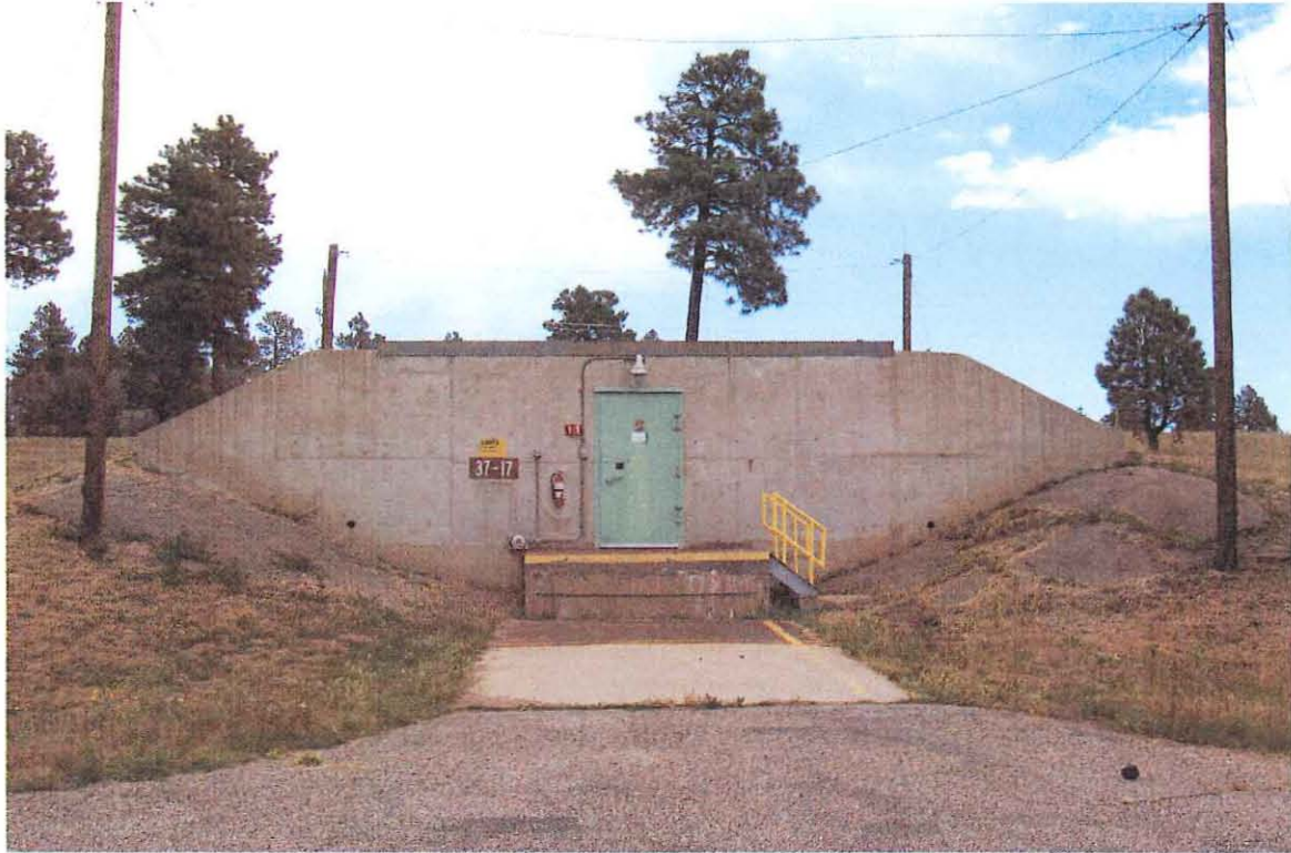
TA-37-17 Southwest Elevation
