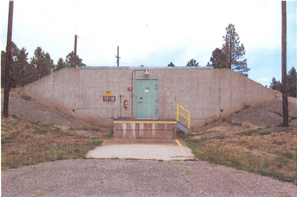
TA-37-18 South Southwest Elevation
