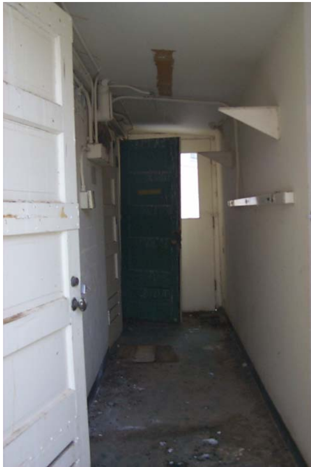
Figure 7a. Interior TA-8-3, enclosed dock
