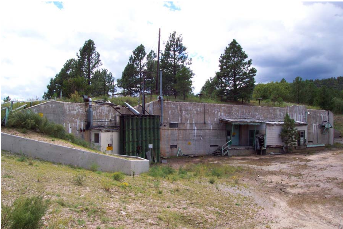
Figure 5d. Exterior of TA-8-1, center right, and TA-8-3, left
