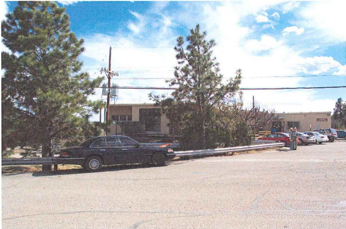
TA-8-21, North side
