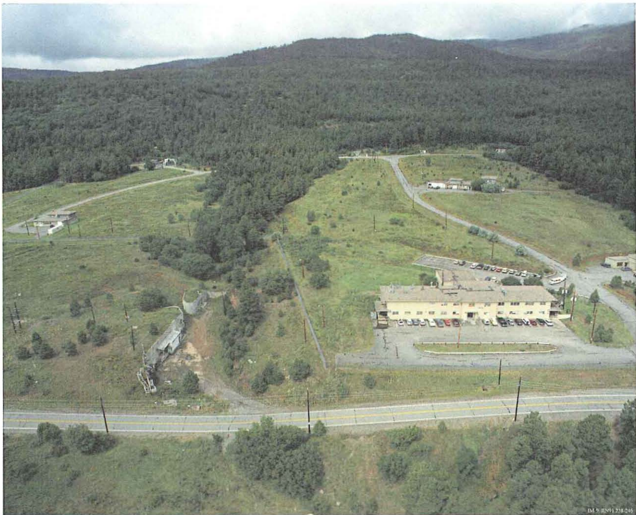
Figure 1. 1991 Aerial of TA-8
