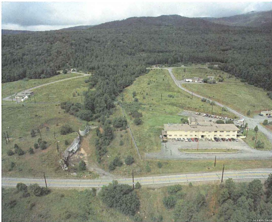
Figure 6. 1991 Aerial of TA-8
