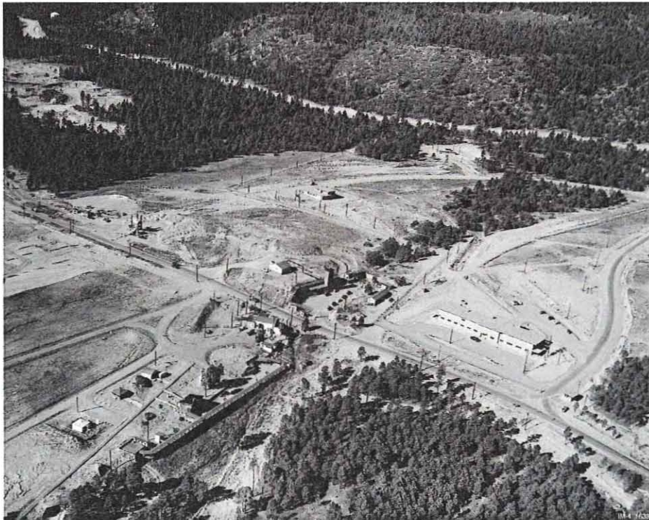
Figure 7. Old TA-9, below road in lower half of photo (1950)
