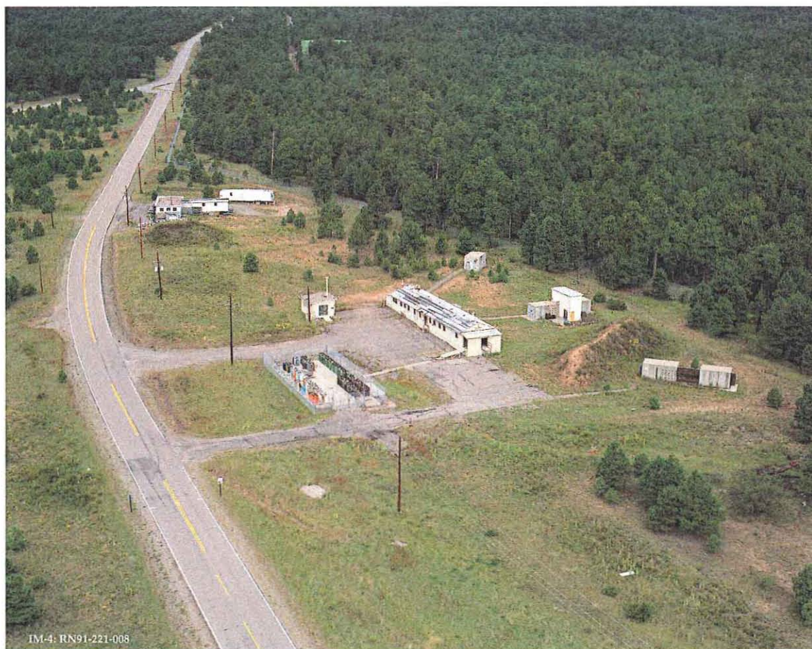
Figure 3. TA-6 WWII Facilities (1991)
