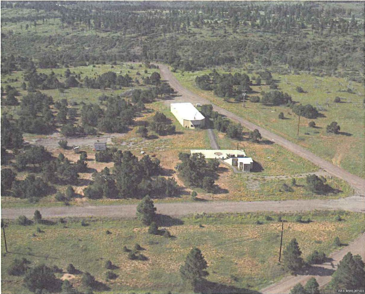
Photo 16. HAZMAT Area LANL IM-9 Photography, Neg. # RN91-207-011 (1991)
