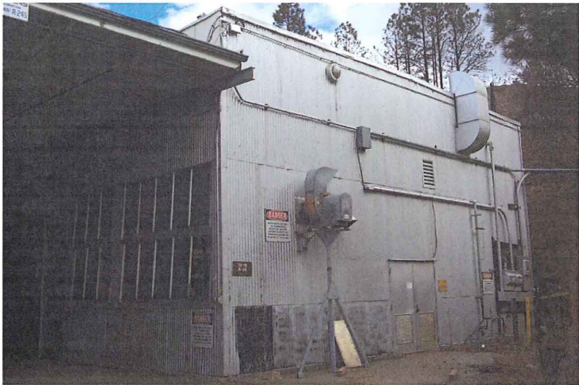
TA-15-20, west side and south side (front), direction northeast.
