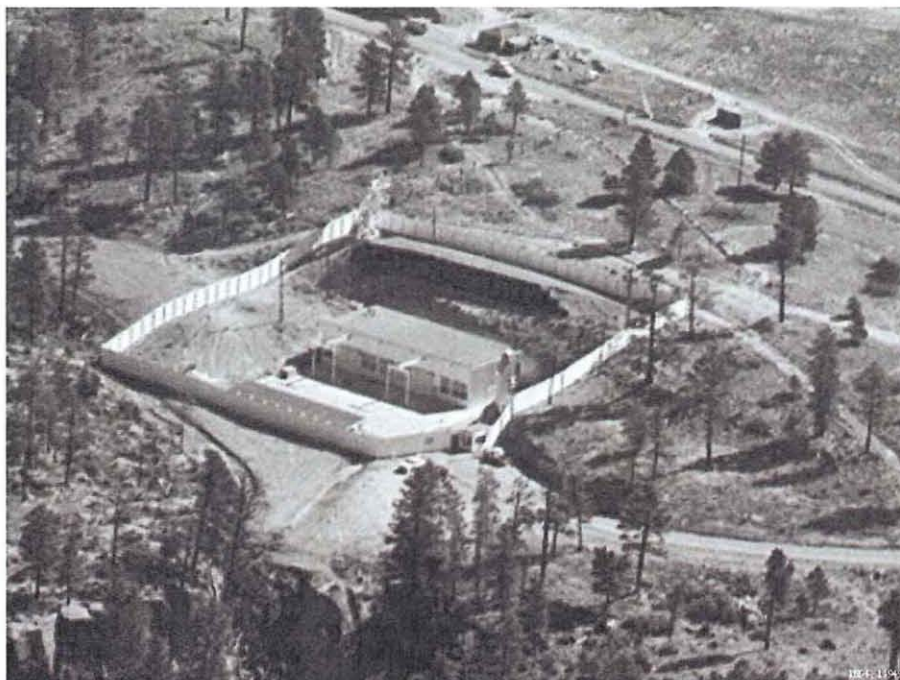
Close up view of explosives assembly building, TA-15-20 (center), and building TA-15-50 (roof visible at lower left side of “no peek” fence area), circa 1950
