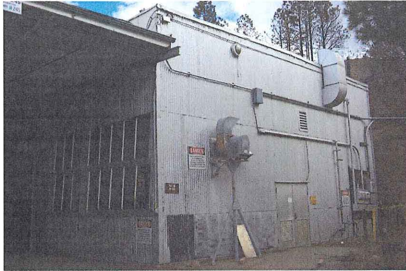
TA-15-245 (covered passage at left) and TA-15-20 (at right)
