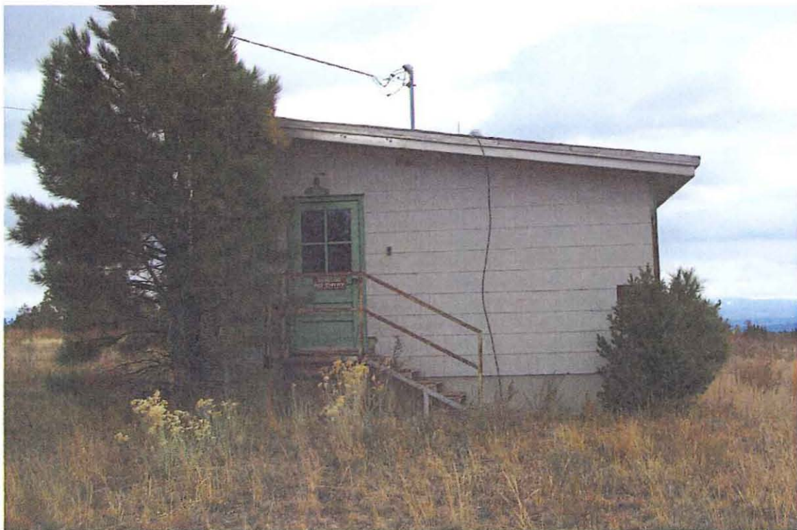
TA-15-23, west side, direction east.
