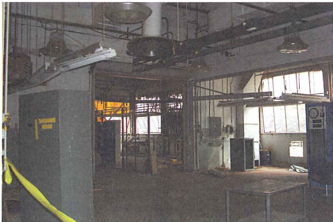
TA-15-20, room 102 looking into room 101, direction northeast.
