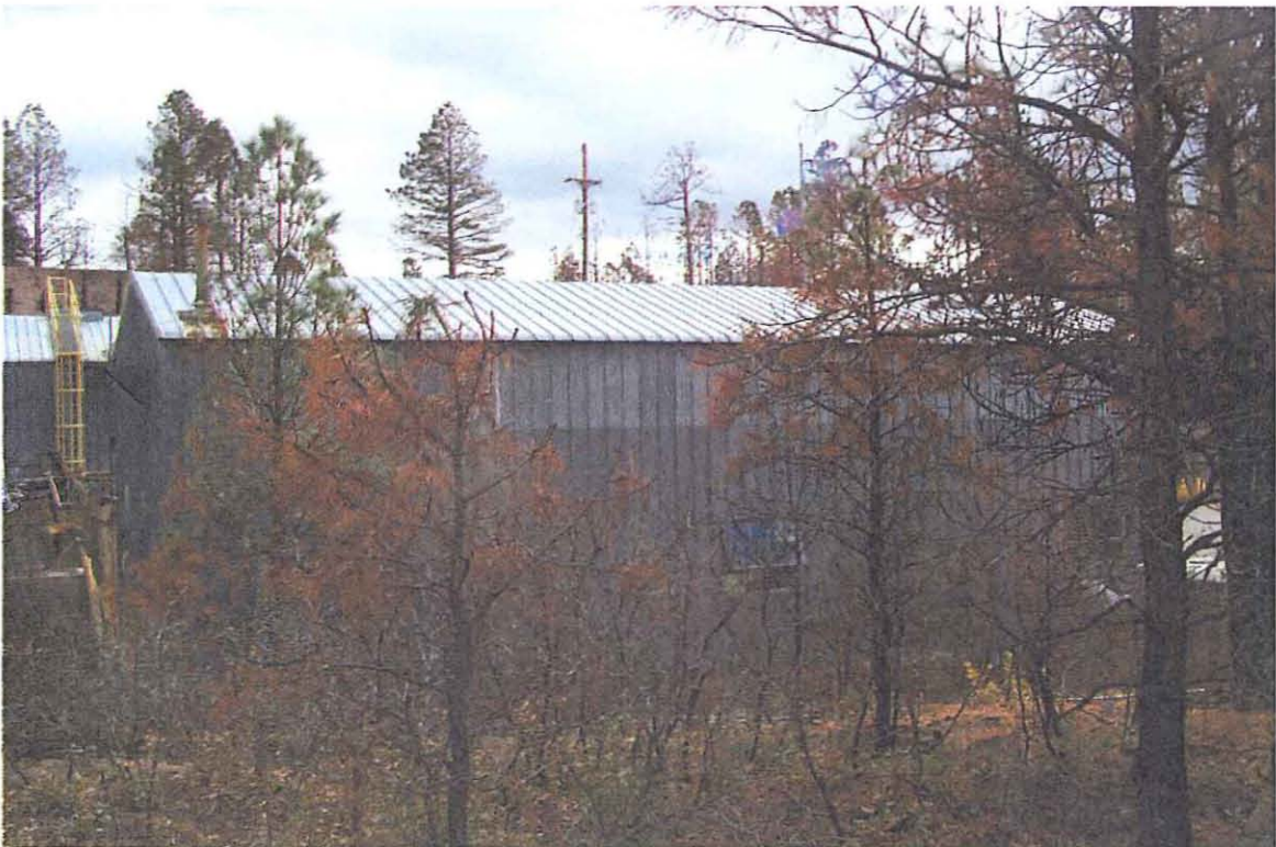
TA-15-194, west side, direction east southeast.
