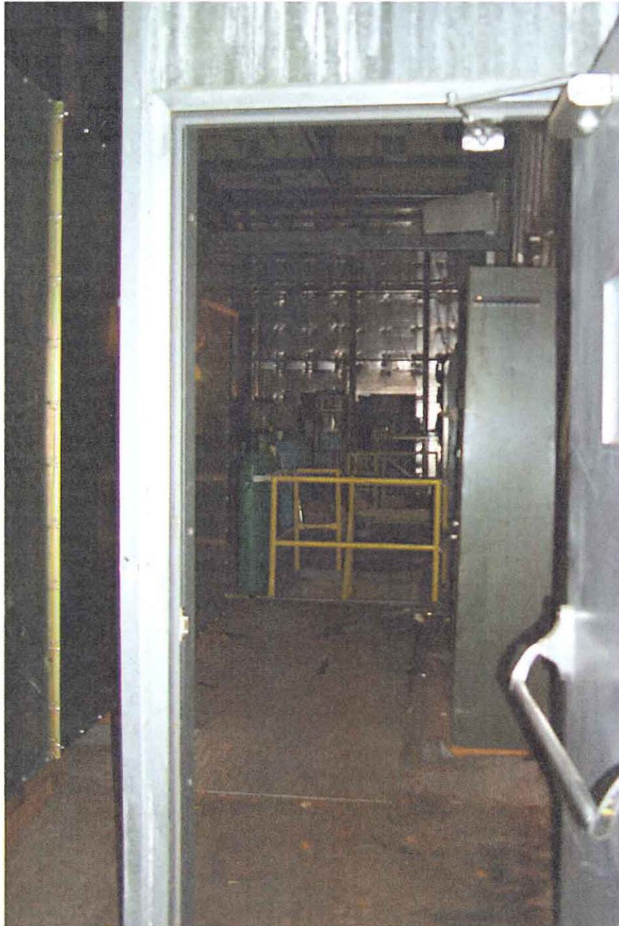
TA-15-245, interior, yellow railing for Pit #1 in center of photo.
