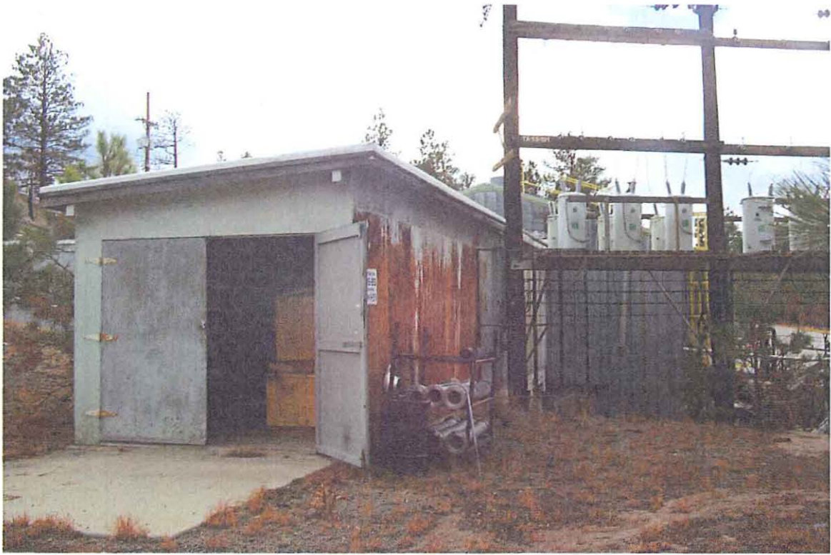
TA-15-213, north and west sides, direction southeast.
