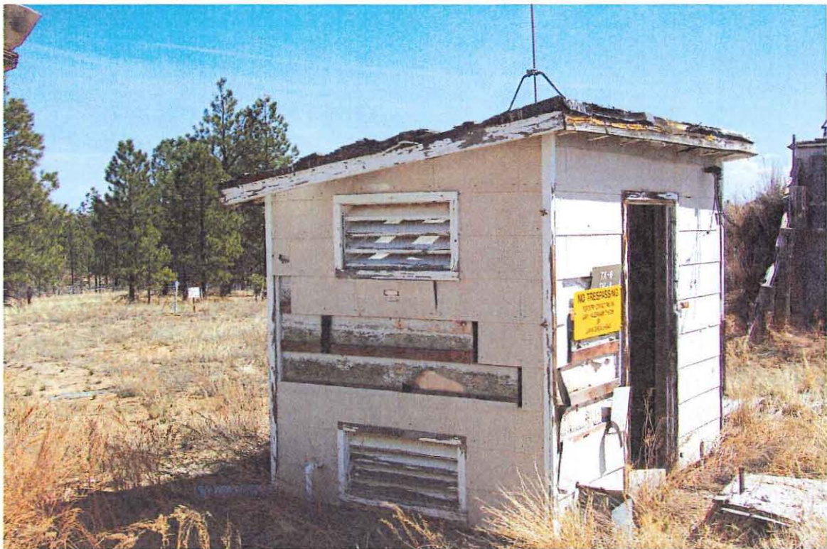
TA-6-2, West and South Elevations
