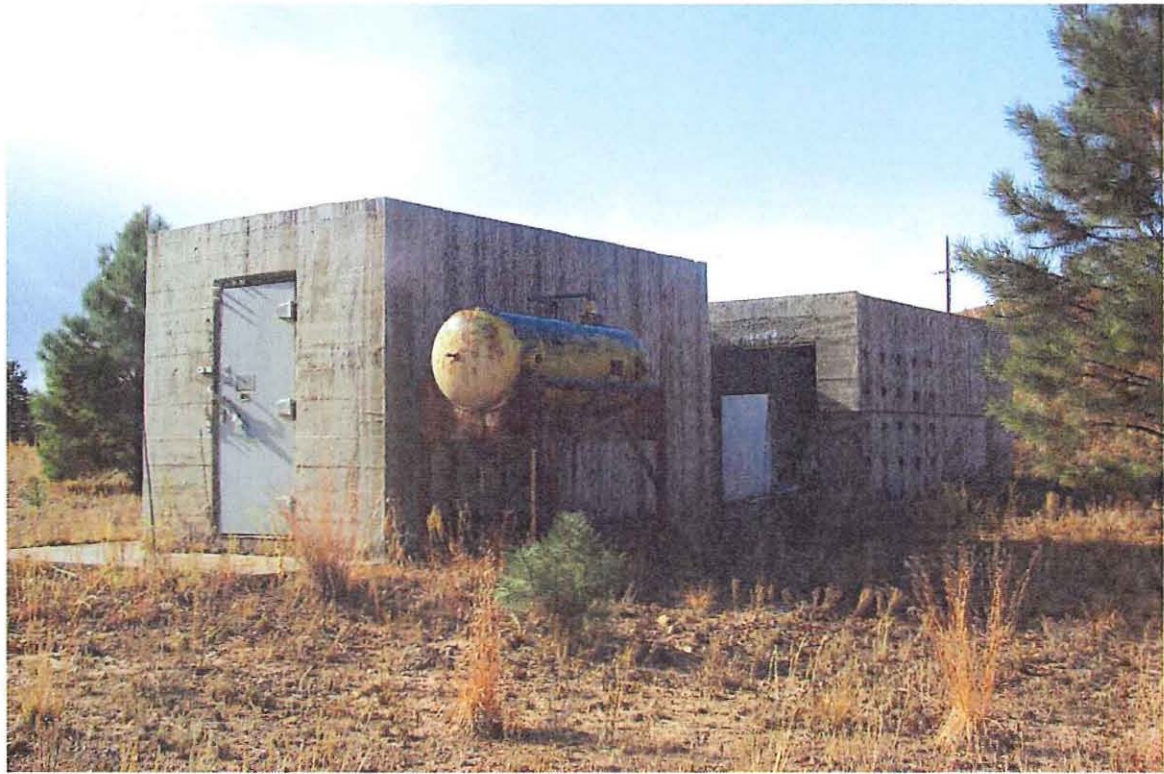
TA-6-9, Northeast and Northwest Elevations
