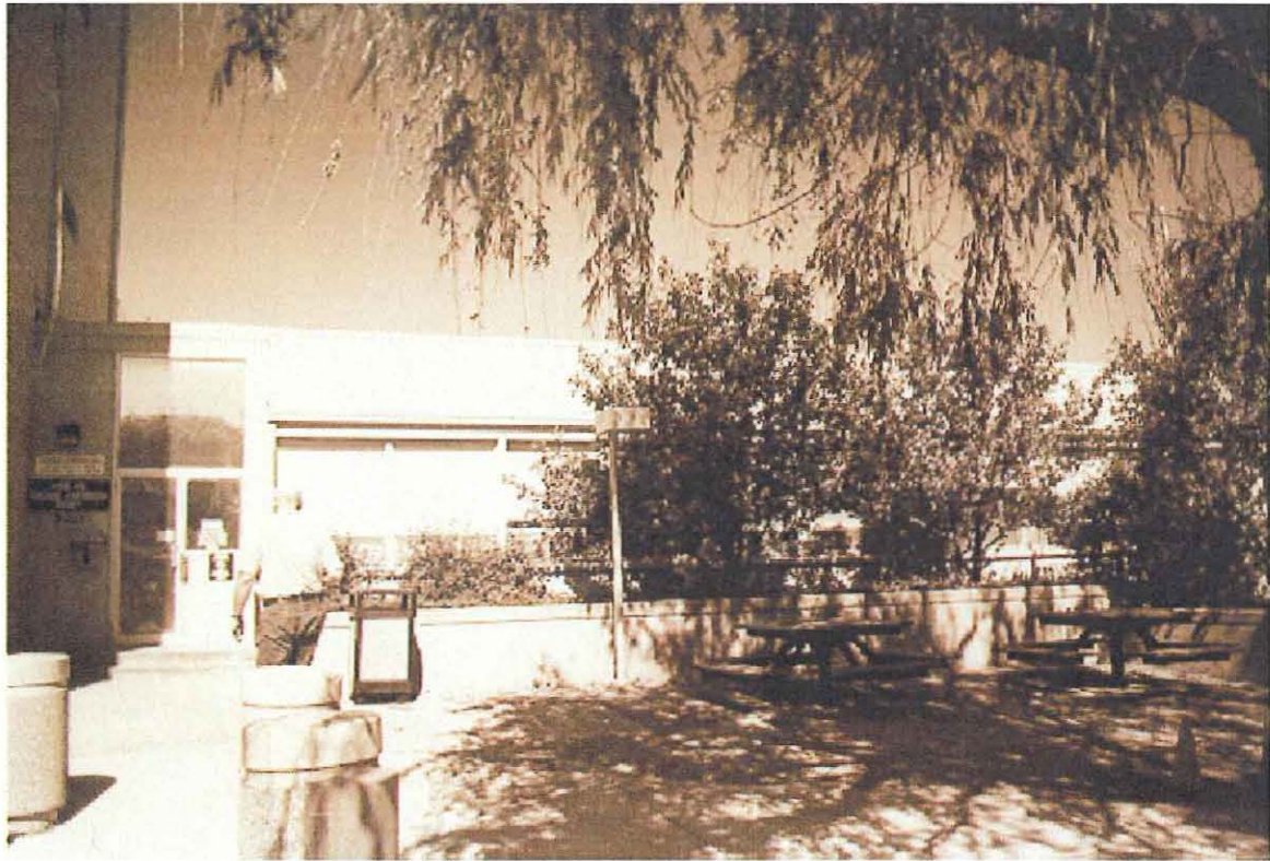
Sherwood Building, TA-3-105, east side (front), direction west
