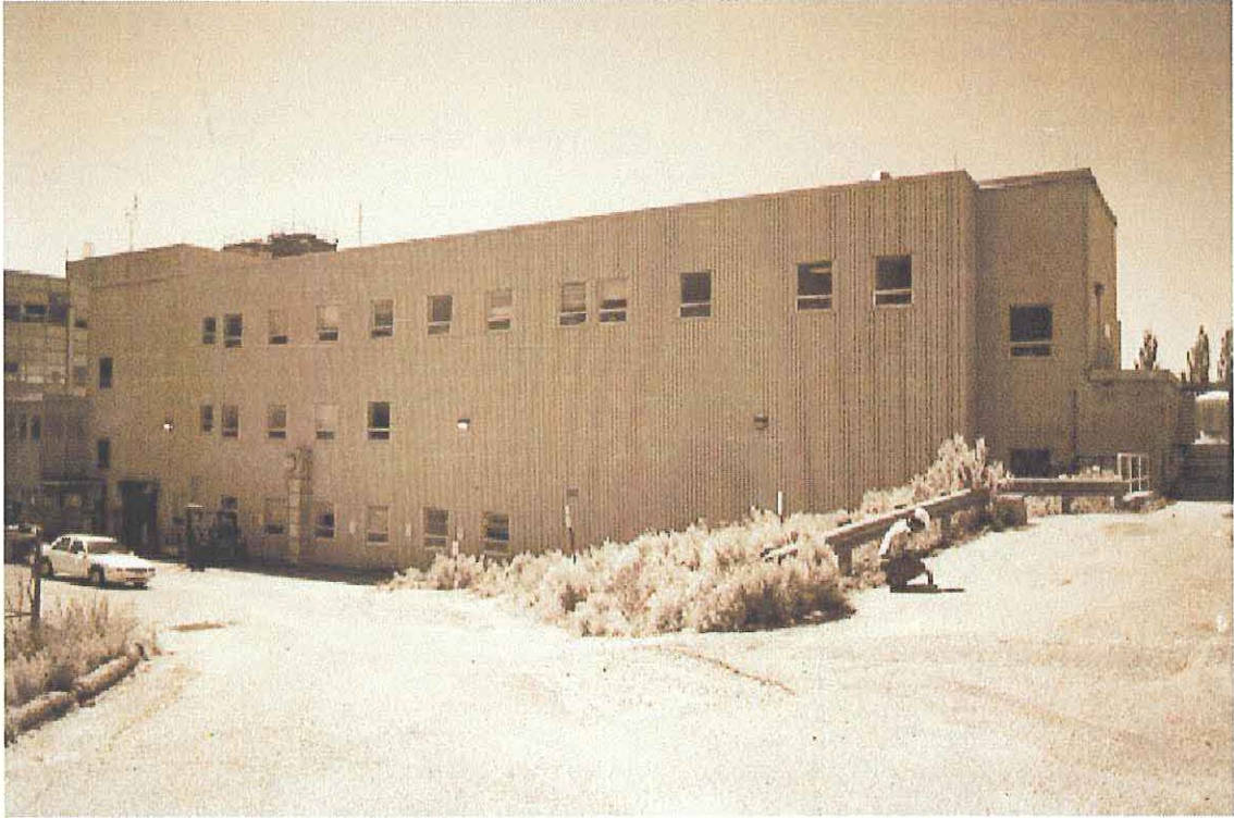
Scyllac Building, TA-3-287, north side, direction south southeast
