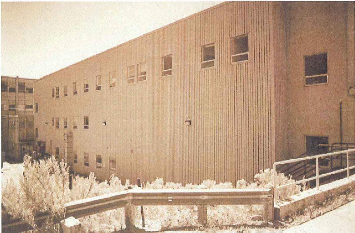
Scyllac Building, TA-3-287, north side, direction southeast
