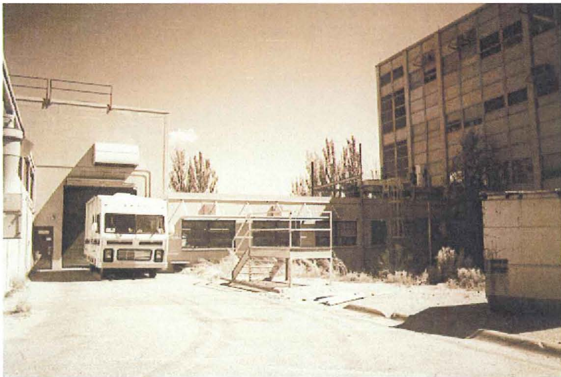
Sherwood Building, TA-3-105, south side, direction north
