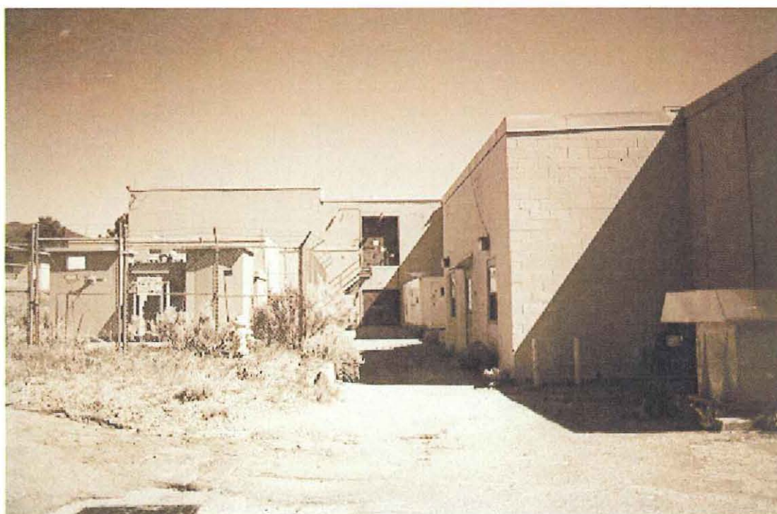
Sherwood Building, TA-3-105, south side, direction north
