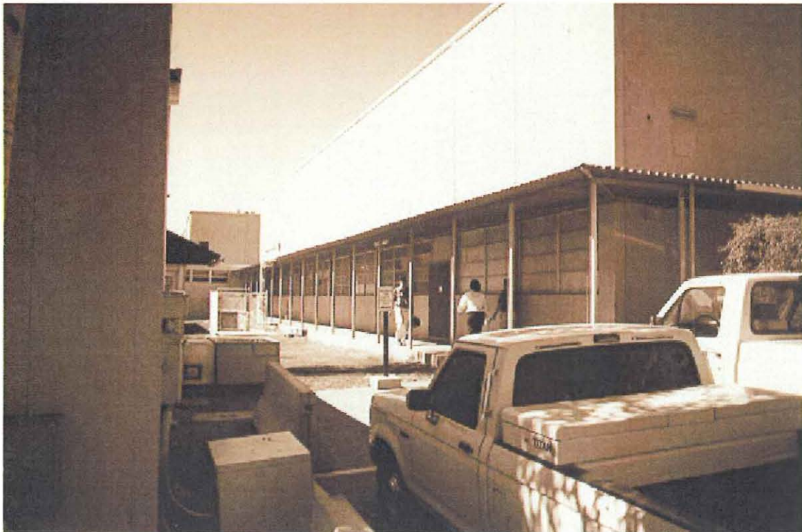
Sherwood Building, TA-3-105, east side, direction southwest
