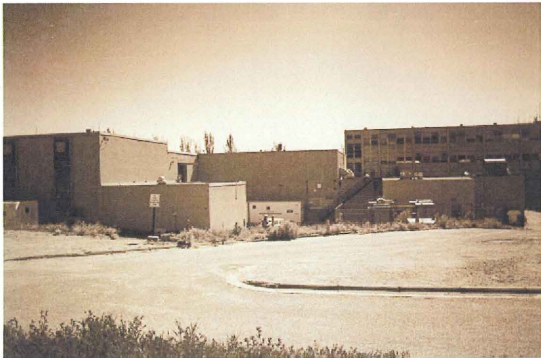
Sherwood Building, TA-3-105, west side, direction northeast
