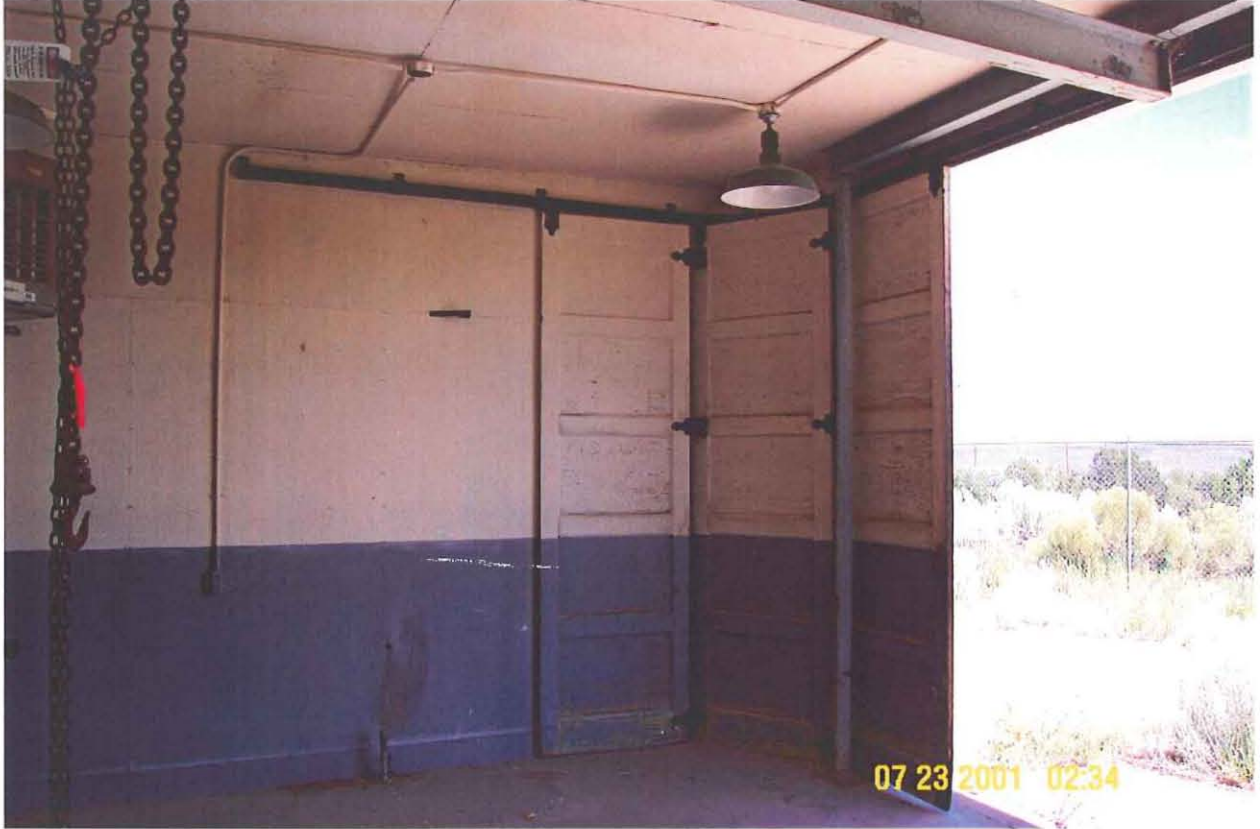
TA-33-40 Interior Sliding Section Door looking southeast
