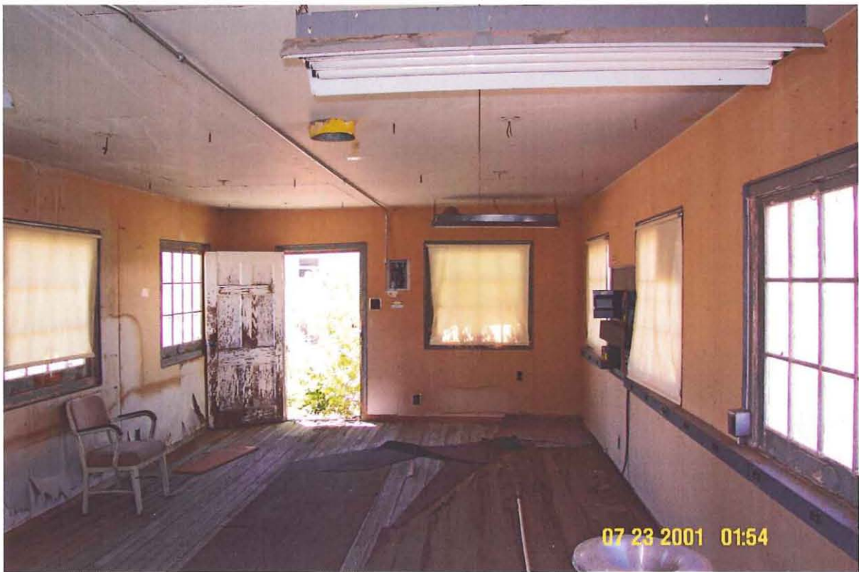
TA-33-1 Interior looking West
