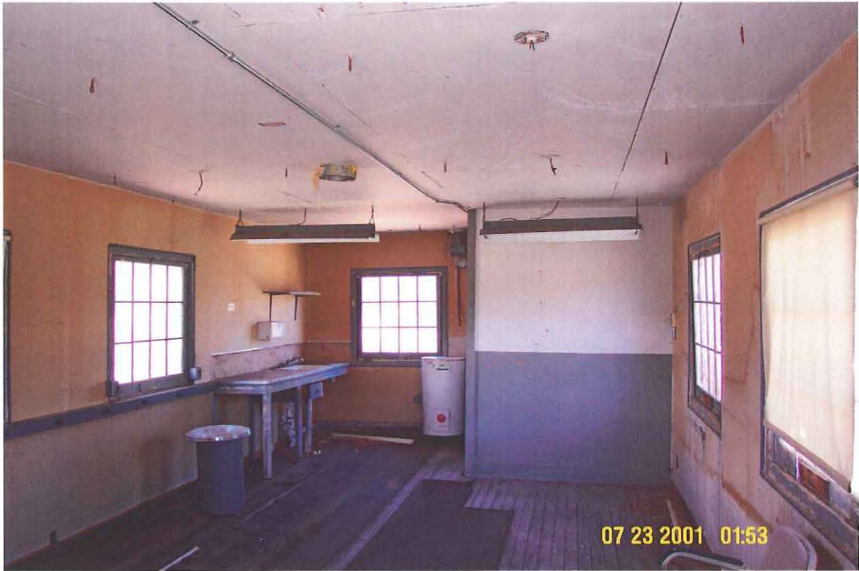
TA-33-1 Interior looking East
