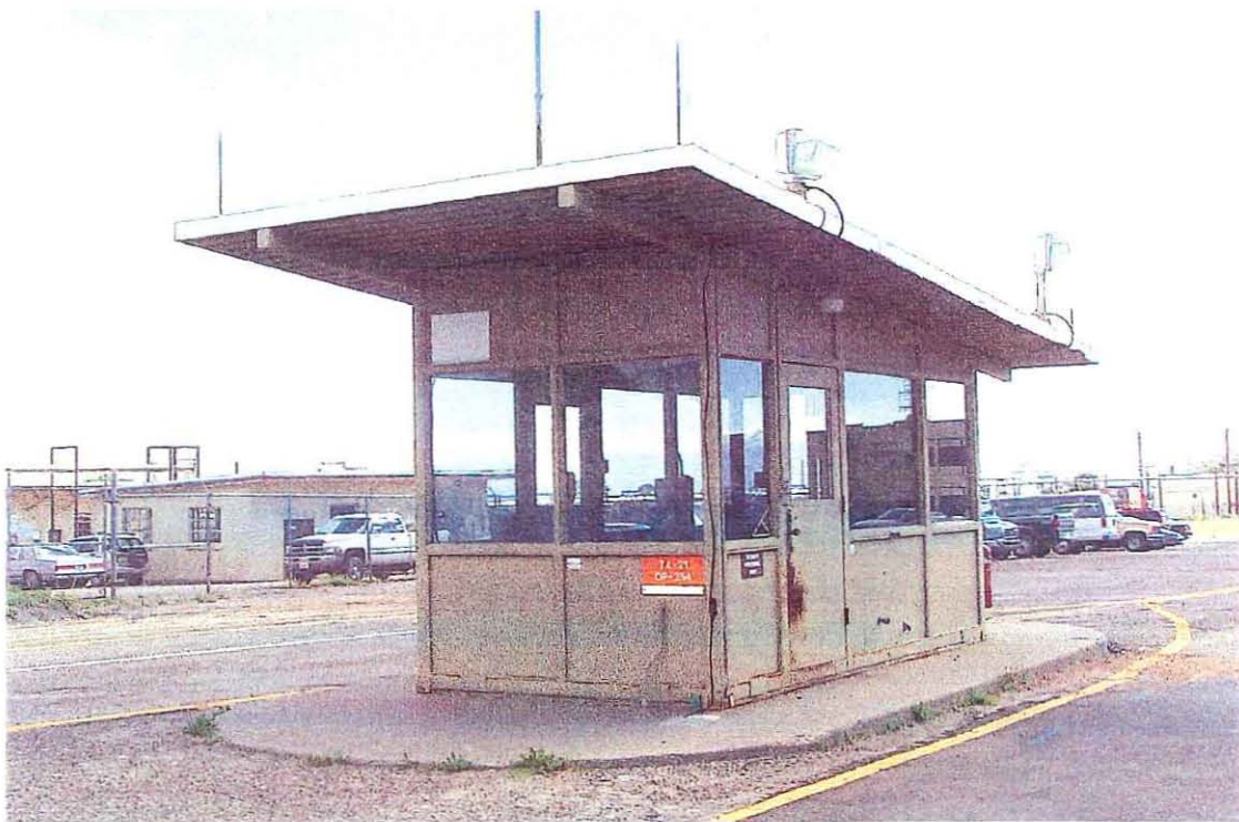
TA-21-254 West and South Elevations
