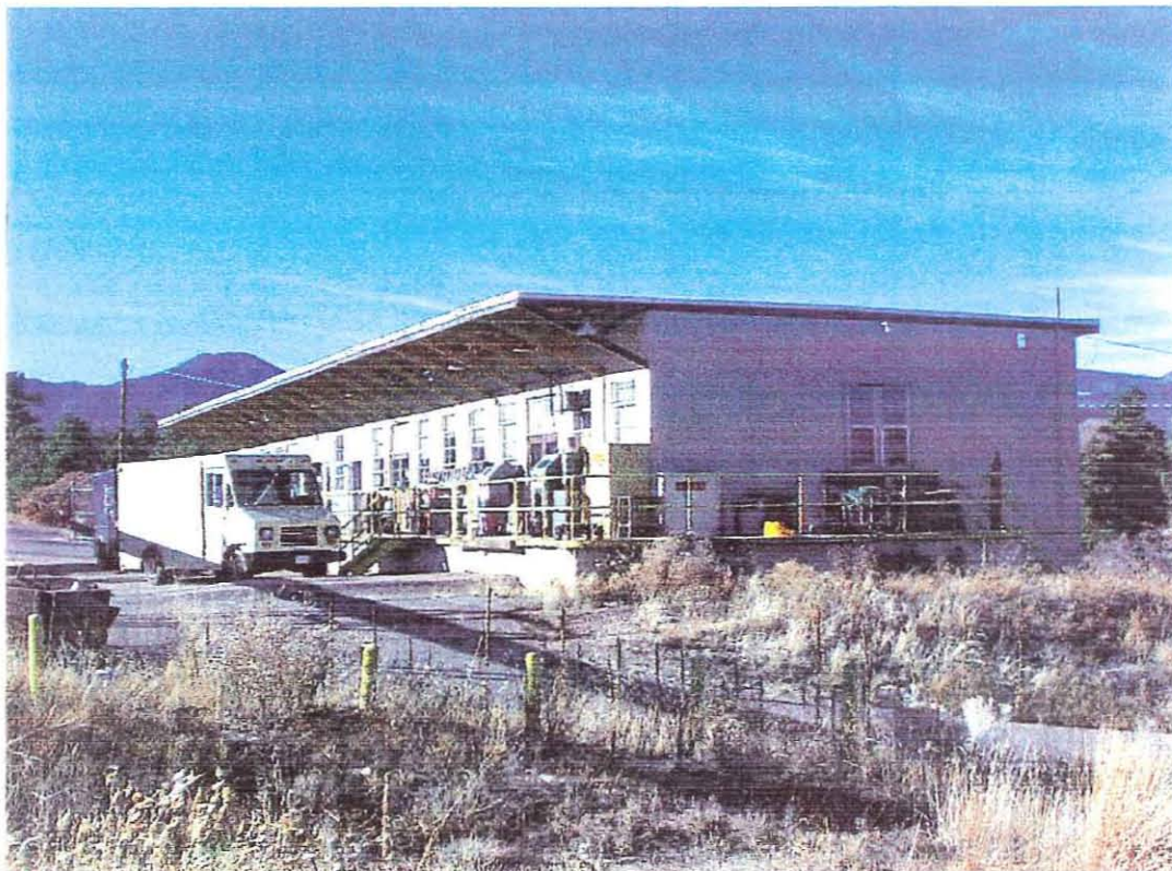
TA-21-31 South and East Elevations
