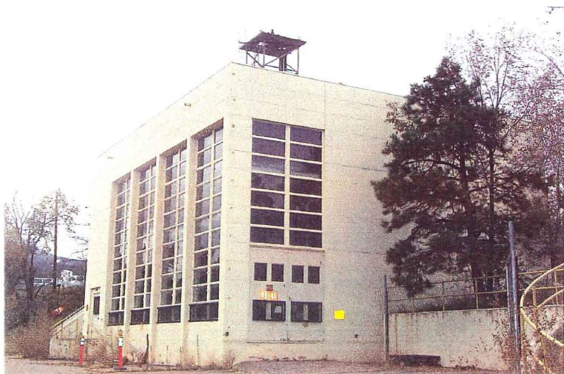
TA-43-41 South and East Elevations
