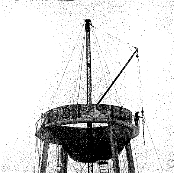
Figure 61. The dismantling of the tank, 1966.
