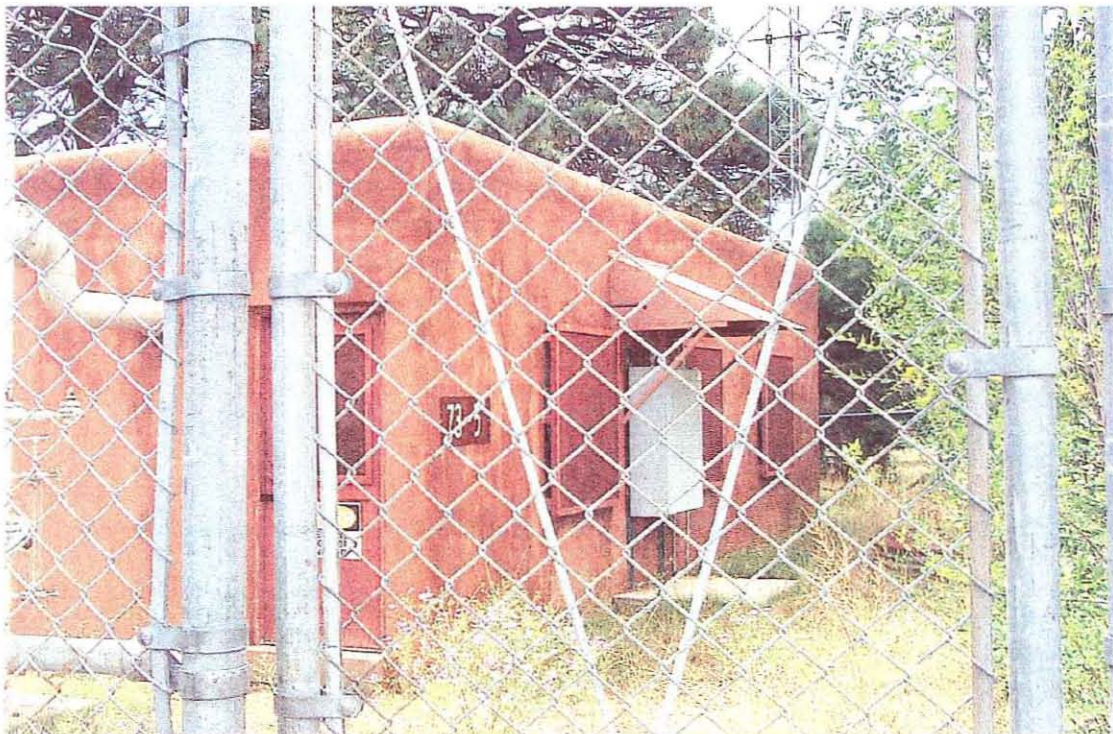
TA-73-5 East and North Elevations
