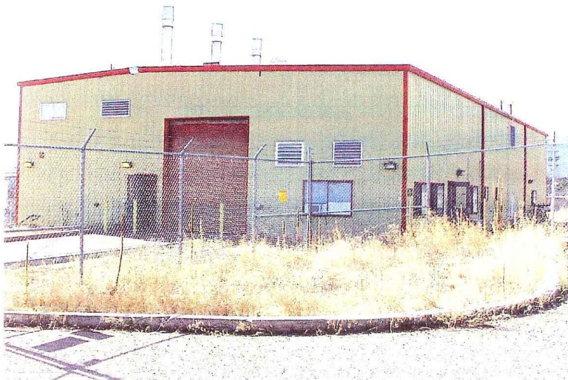
TA-21-357 East and North Elevations
