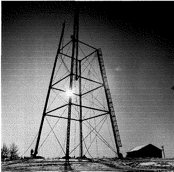
Figure 62. Dismantling the tower.
