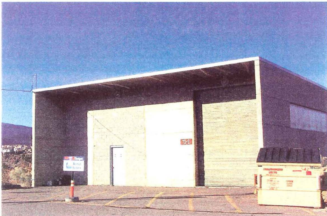
TA-73-2 South and East Elevations
