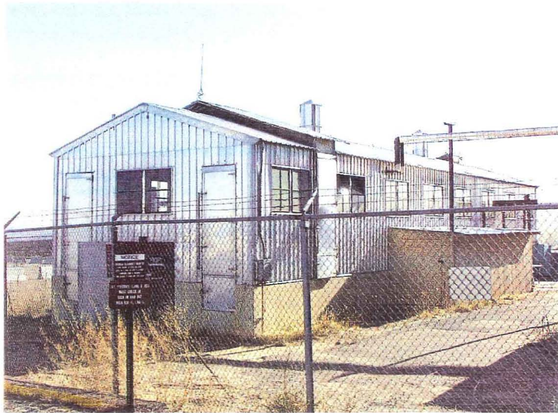
TA-21-46 North and West Elevations
