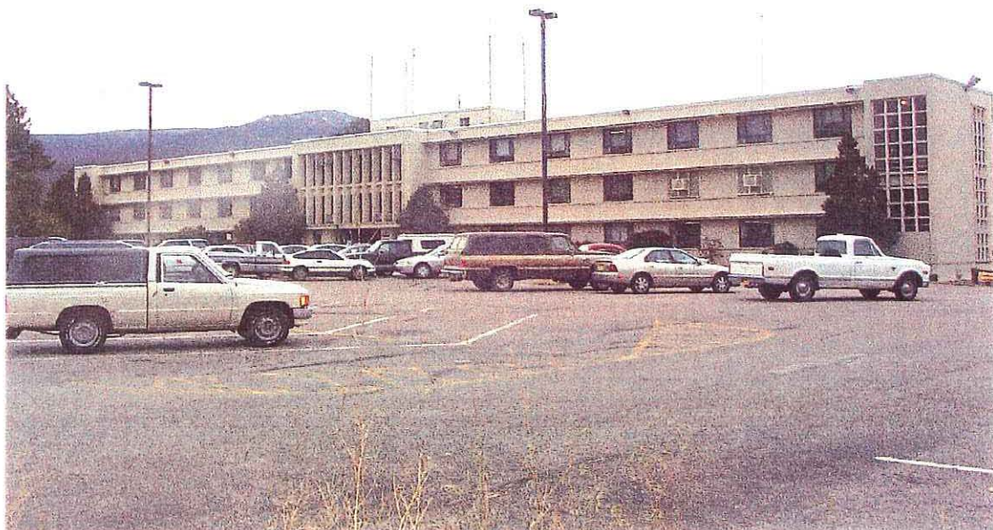
TA-43-39 South and East Elevations
