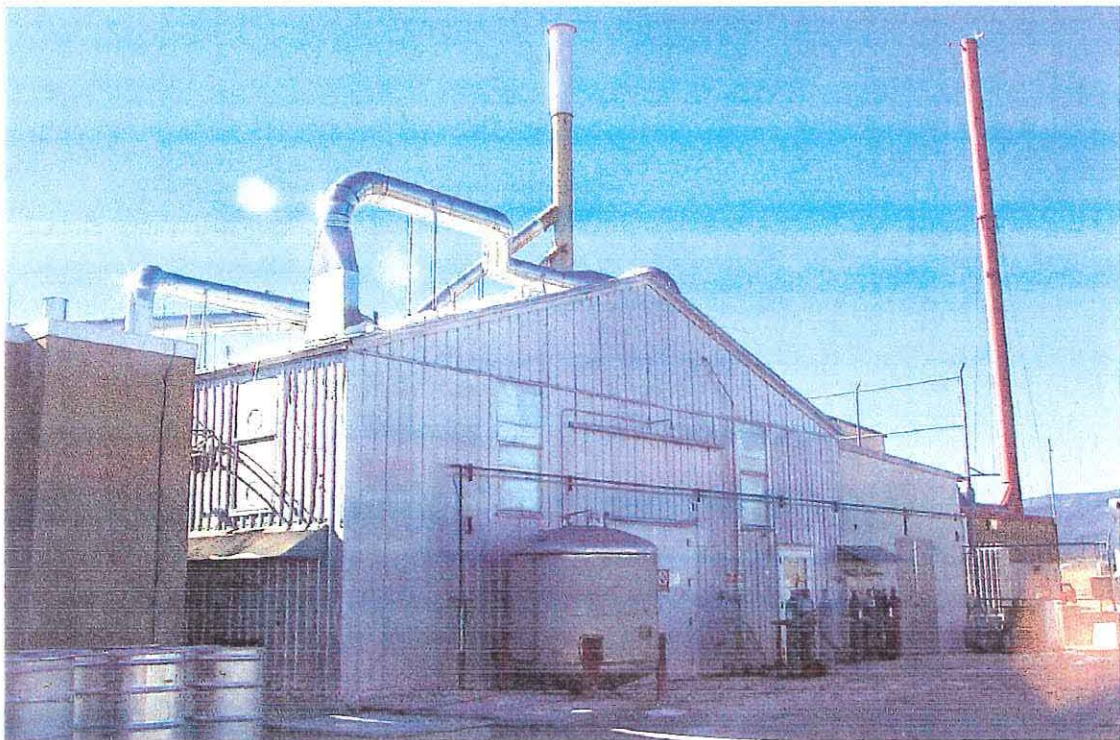
TA-21-152 East and North Elevations
