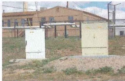
Telephone Pedestals/Cabinets
