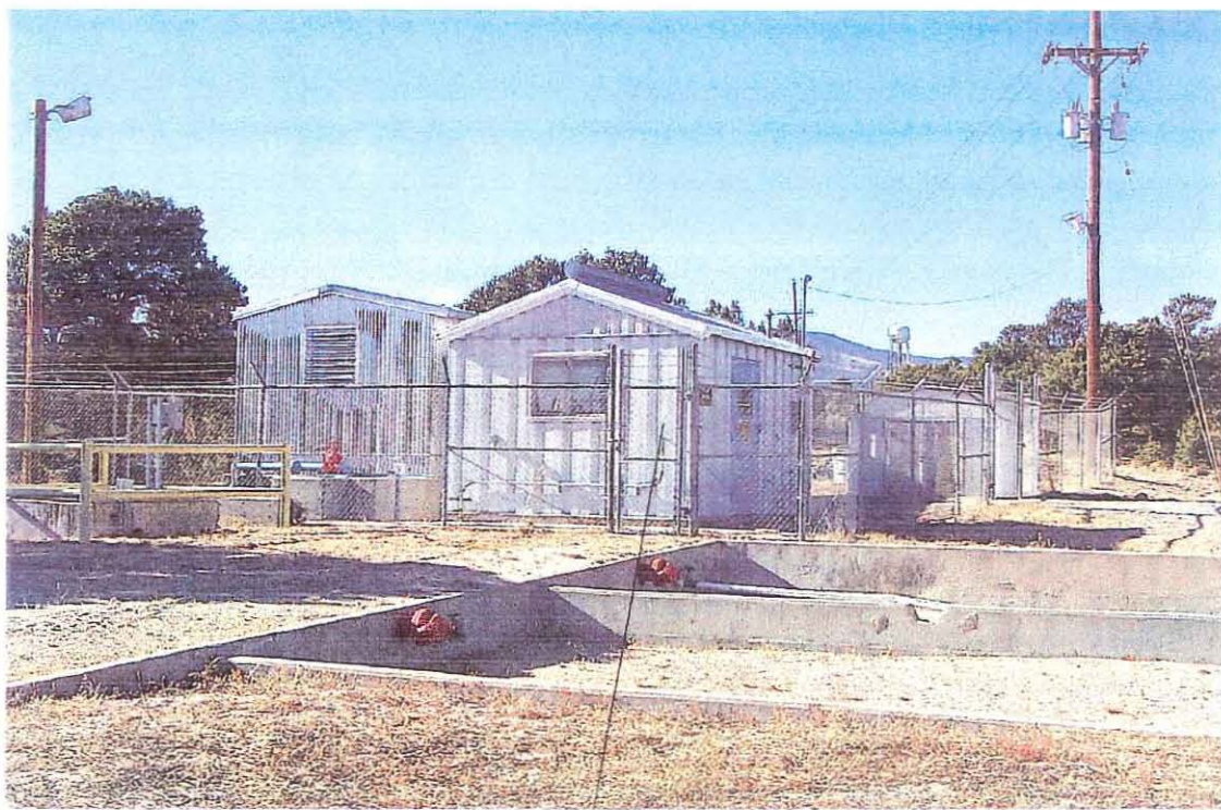
TA-21-229 East and North Elevations
