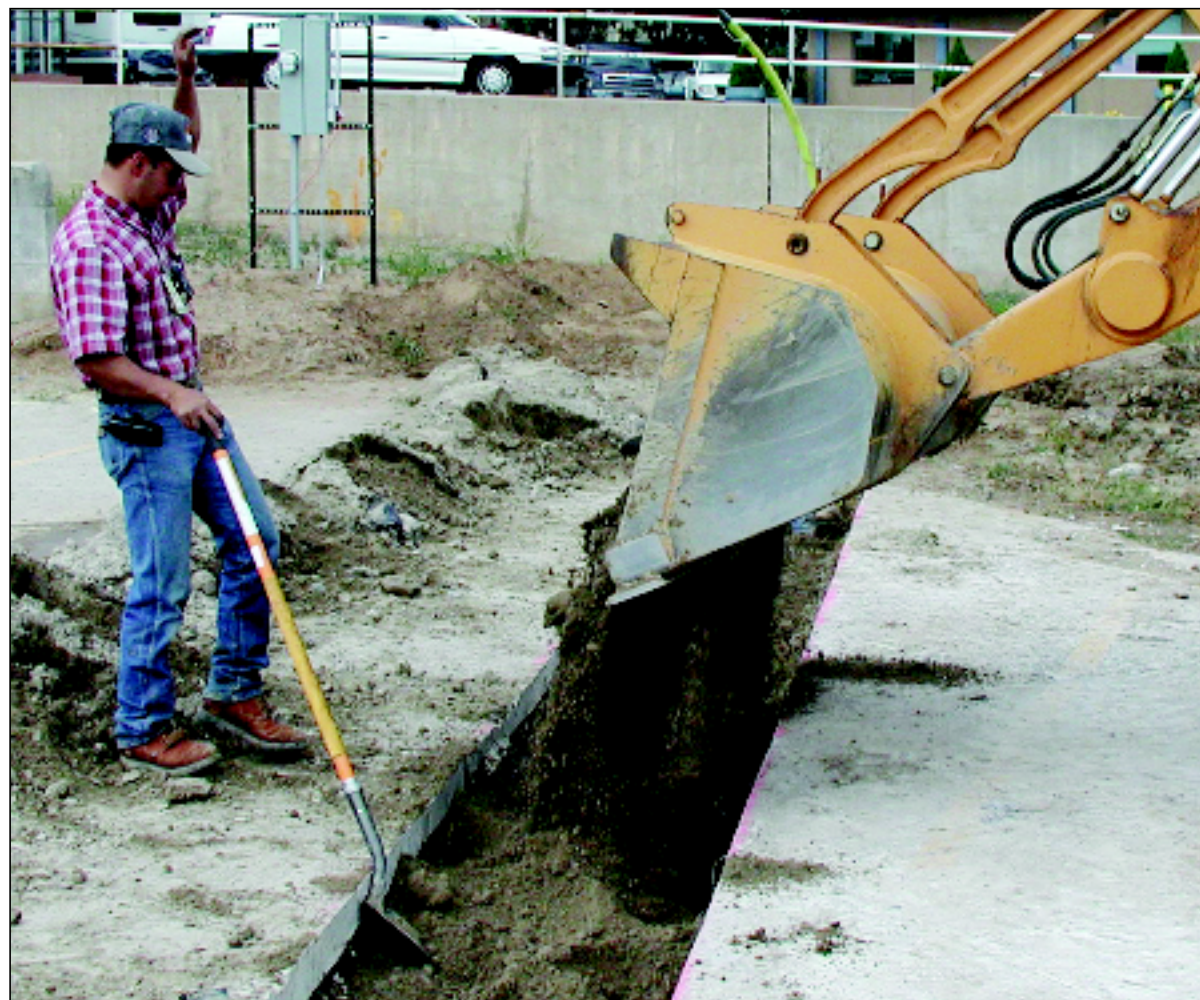
The Laboratory is reconditioning the soil underneath the Knights of Columbus parking lot using a process known as soil vapor extraction, which removes contaminants from the existing soil. In the photo, Joe Sena of Los Alamos Technical Associates, a remediation subcontractor, directs the bedding and back-filling of a soil vapor extraction well piping trench. During the Manhattan Project, the site was used as a fuel tank farm and drum storage yard where a combination of fuel and oil was spilled.
