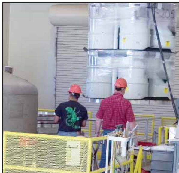
Fourteen 55-gallon drums of plutonium-239 sealed sources are bundled in two layers and wrapped in strips of heavy plastic, ready to be loaded into a TRUPACT-II container at Technical Area 54. The sealed sources recently were delivered to the Waste Isolation Pilot Plant near Carlsbad. Paul Apodaca, left, of the Nuclear Waste and Infrastructure Services (NWIS) Division and Mitch Carter of Carlsbad Operations (EES-12), supervise the loading as the waste drums are hoisted in the air and moved to an open TRUPACT-II. Photos by Patricia Leyba, Environmental Stewardship (ENV) Division
