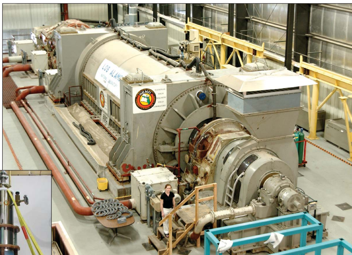
Shown above is the 1.4 GVA generator. It can deliver 750 mega joules of energy to the magnets at the National High Magnetic Field Laboratory. It was used to power the 60T long-pulse magnet before the magnet's failure and will power both the 60T rebuild and the 100T magnet, both still in production. The inset photo is the 50T mid-pulse magnet. This mid-pulse magnet is used for high precision magnetotransport and optics measurements. Above photo by Kevin Roark; inset photo by Rebecca E. McIntosh, NHMFL.
