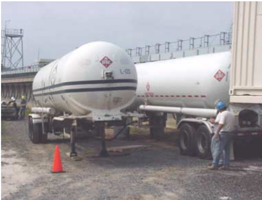
Figure 3 - Propane tankers parked on east side of tank.
