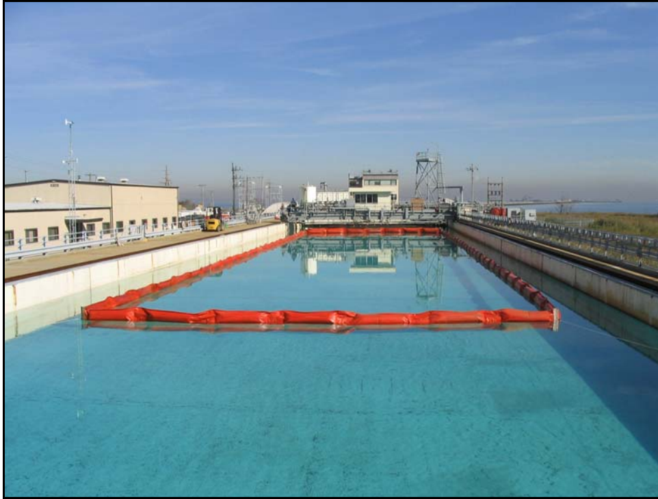
Figure 2-1: Ohmsett Test Tank with Containment Boom, October 2003.
