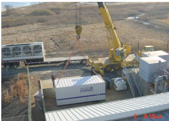
Unloading the large industry chiller for the test tank.
