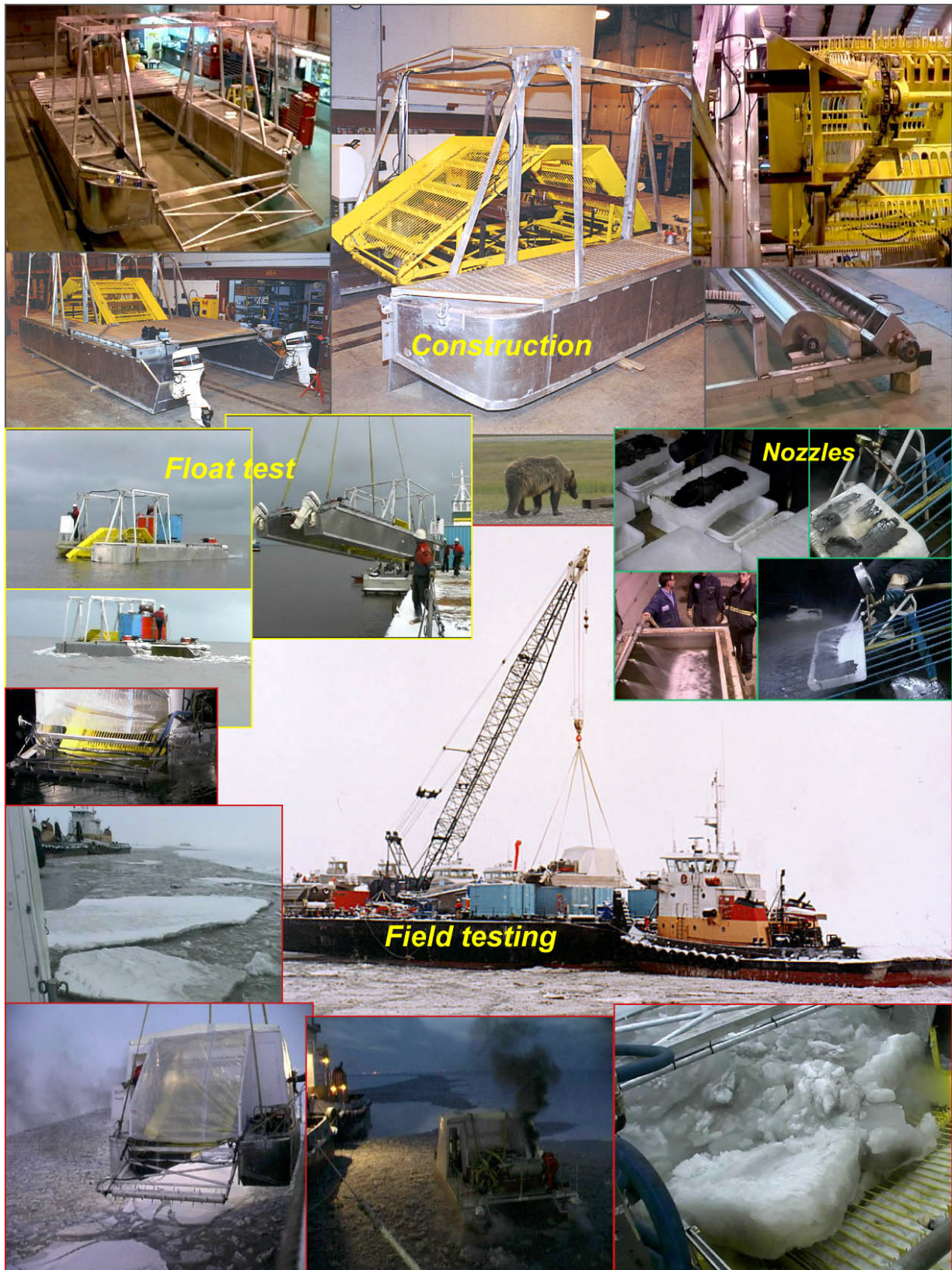
Figure 2.4 Photos from Phase 4 construction and field testing in Prudhoe Bay, Alaska.
