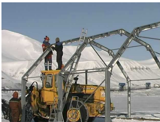
Assembling the 9m x 18m tent on the ice.
