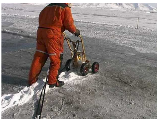
Chainsaw mounted on wheels gives excellent control and cutting speed.
