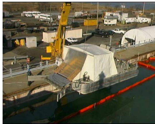
Work platform being crane lifted into the tank during preparations.
