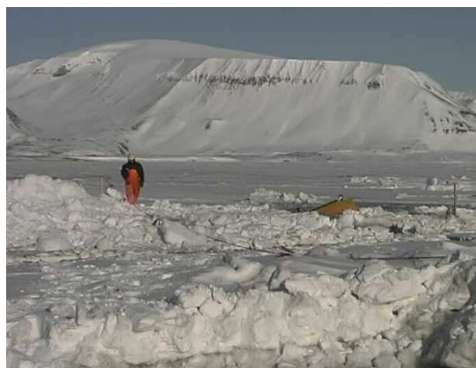
Only a small part of the excavator visible just after it went through the ice and sank.
