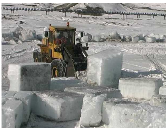
Nearly 500 metric tons of ice was moved away to reduce the load on the floating ice.
