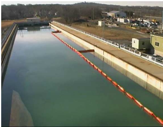
Boom installed at the west wall of the tank.
