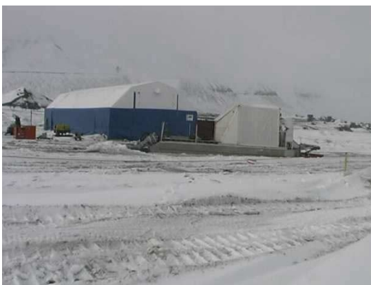
Work platform in pool outside tent.
