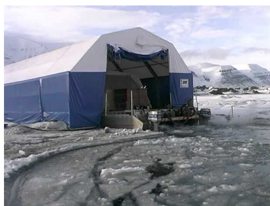
Work platform moving into the tent.
