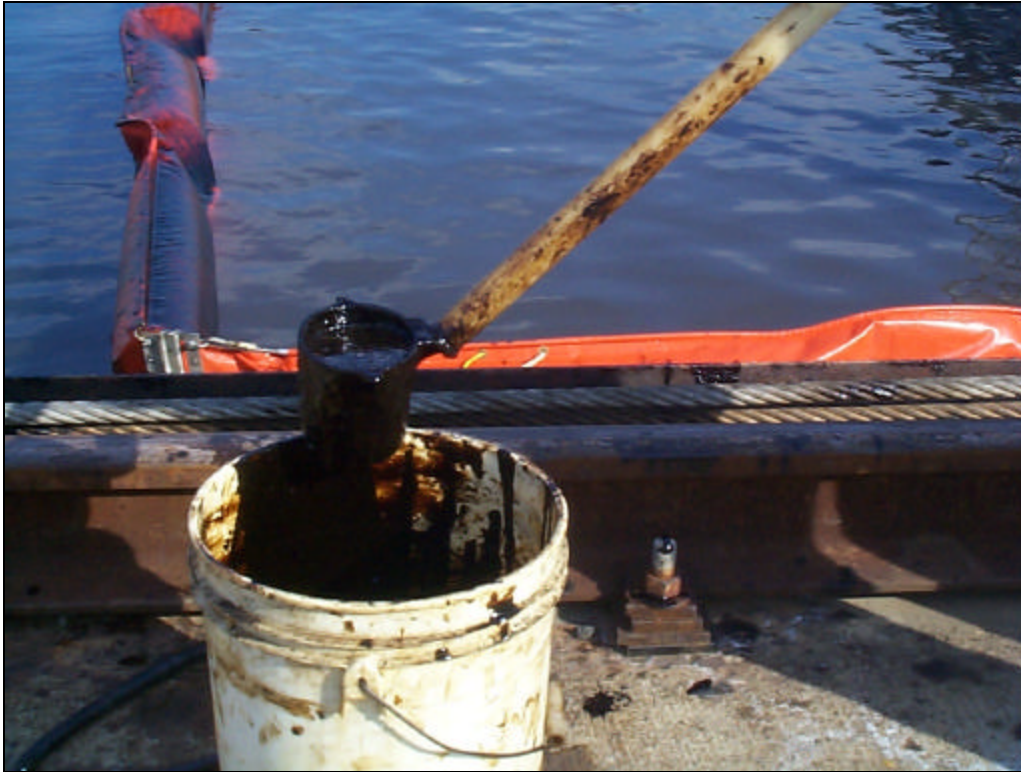
Figure 10. Ladle Used to Remove Oil Herded to Corner of Containment Boom
