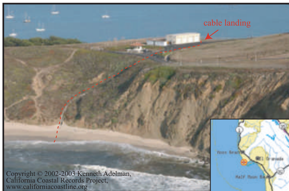
Figure 4: A photograph looking south showing the shore landing of the ATOC/Pioneer Seamount cable. Note inset map showing the photograph location in northern Half Moon Bay, California. The red dashed line represents the location of the cable that is within an underground conduit that parallels the drainage ditch. The cable is buried below the beach (Howe 1996).
