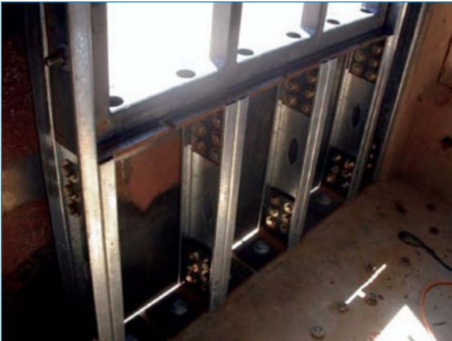
Figure 3-12: Metal stud blast wall.
