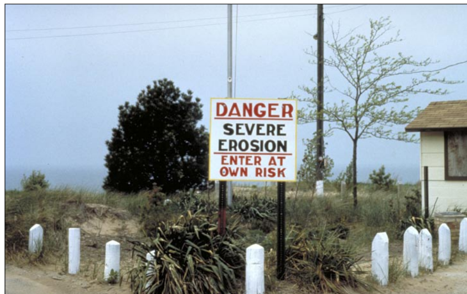
Figure 26. Erosion at Oval Beach, Saugatuck, Michigan. Photo credit: Michigan DNR, Land and Water Management Division, Coastal Programs Unit, from the EPA Great Lakes web site.
