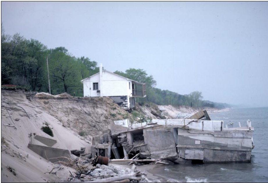
Figure 28. Shoreline erosion - house in shambles, Ogden Dunes Indiana. Photo courtesy of Carole Y. Swinehart, Michigan Sea Grant Extension, from the EPA Great Lakes web site.
