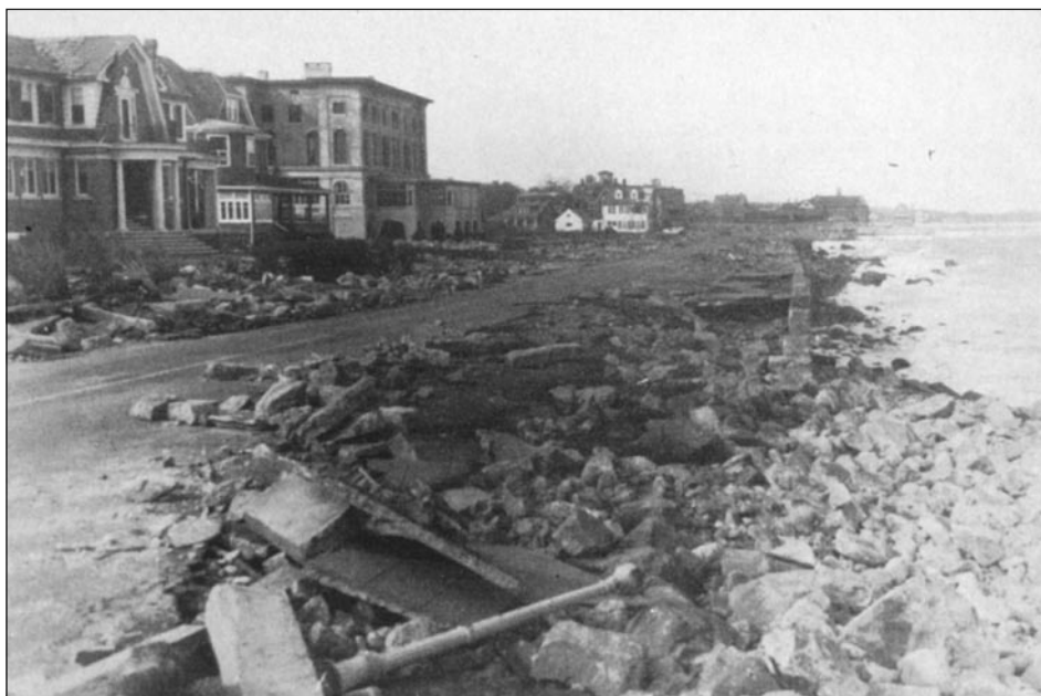
Figure 29. Destruction of the seawall at Narragansett Pier in southern Rhode Island due to the New England Hurricane of 1938. Archival Photography by Steve Nicklas, NOS, NGS, from the NOAA Photo Library.
