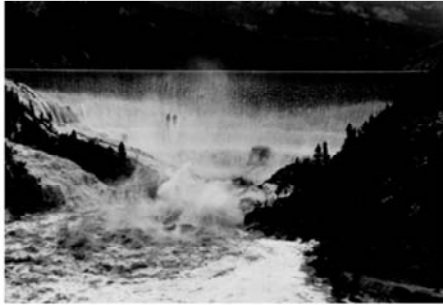
June 8, 1964 20 hour duration 1 m overtopping
