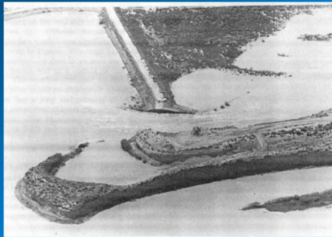
DMAD spillway shortly after failure (1982)
