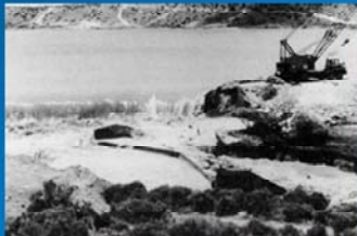
Spillway Breach
