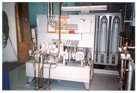
Photo 8 Hydraulic Power Unit with Accumulators
