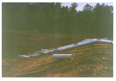
traditional pipe-and-riser spillway systems, generally results in a lake that will fluctuate more as a result of the inherit inefficiency of the siphon until priming occurs. Siphons prime with a head or water surface elevation between 1 and 1-1/4 times the diameter of the siphon above the siphon invert. Once a siphon primes, there is very little increase in outflow as the lake surface rises.
