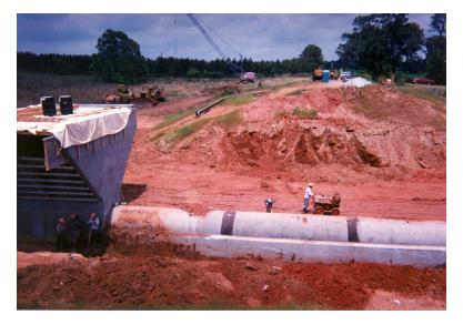
Removing and replacing the existing conduit typically offers the most thorough rehabilitation option for impaired conduits through dams, although this option can be cost-prohibitive.
