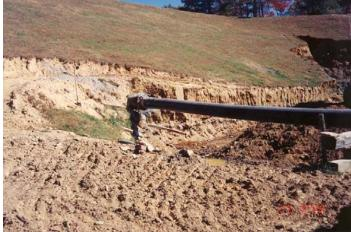
The liner will typically have a roughness value of approximately ½ of the corrugated metal pipe. When designed and installed properly, the slipline technique will add additional years of service life to the existing pipe conduit spillway. A sand diaphragm drain is typically installed around the downstream portion of the existing conduit to limit the potential for soil piping as the CMP eventually corrodes and deteriorates.
