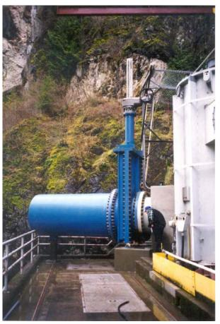
Photo 4 Motor-Operated Jet-Flow Gate
