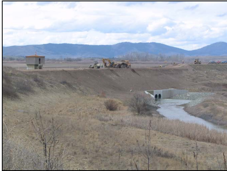
Figure B-58. —Pablo Dam nearing completion.
