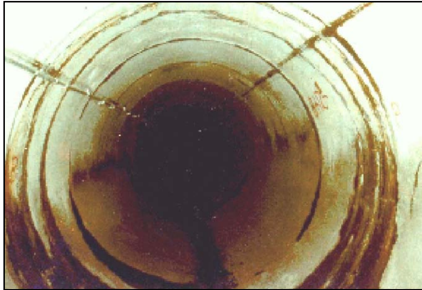
Figure B-66. —View of the interior of the outlet works after grouting.
