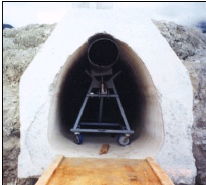
Figure B-53. —Existing 6-foot diameter elliptical conduit.
