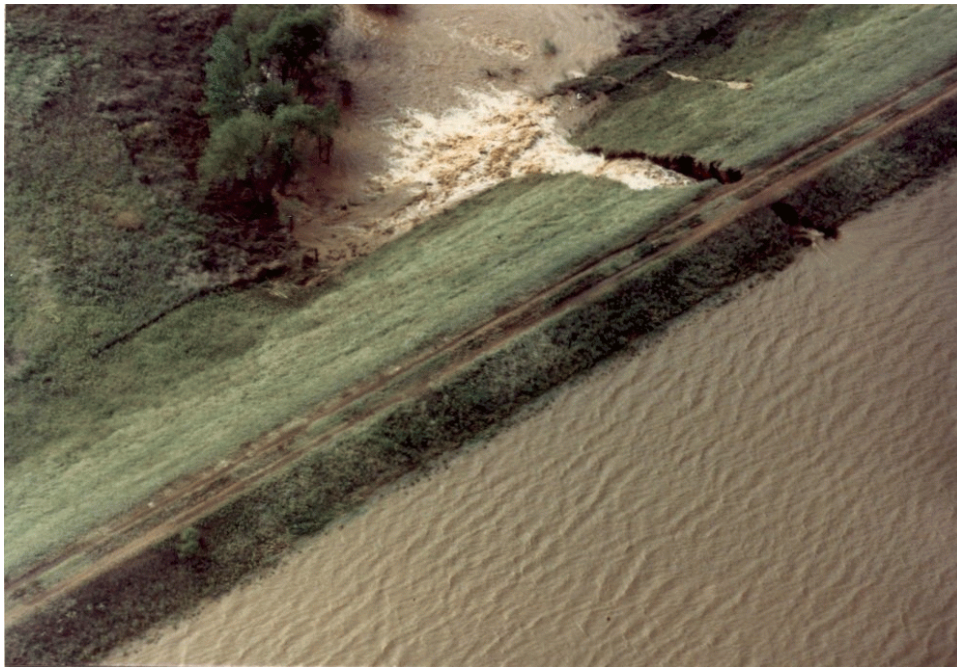
Figure B-77. —Aerial view showing the failure of Upper Red Rock Site 20 Dam.
