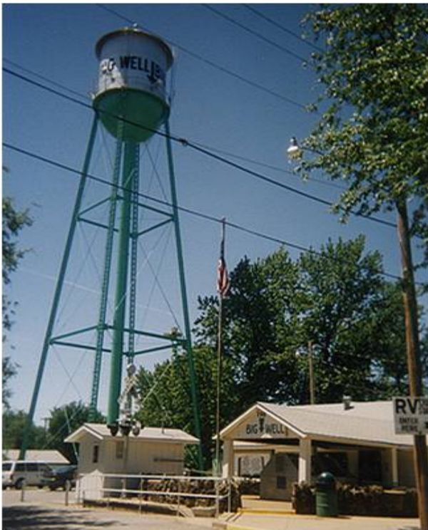
water tower before
