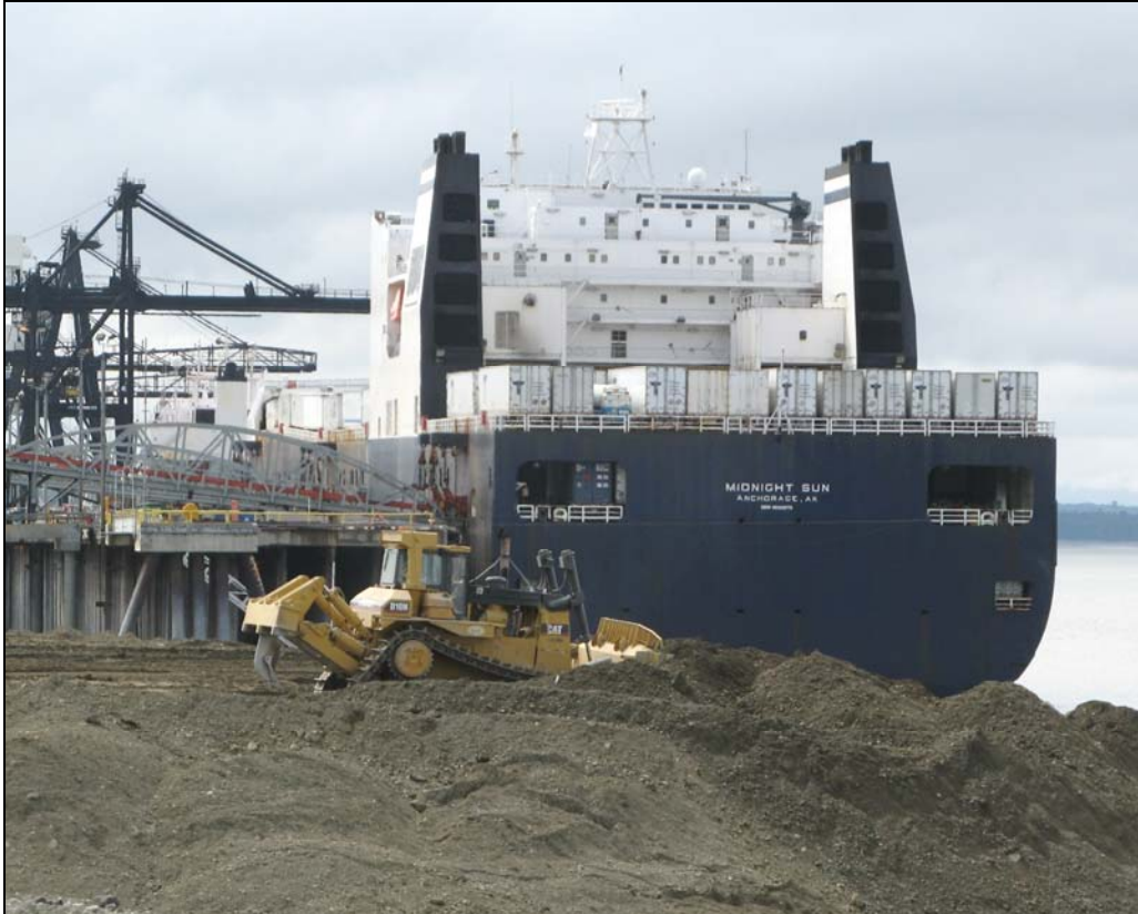
Photo 9. Caterpillar D-10 bulldozer pushing fill into place at the water front.
