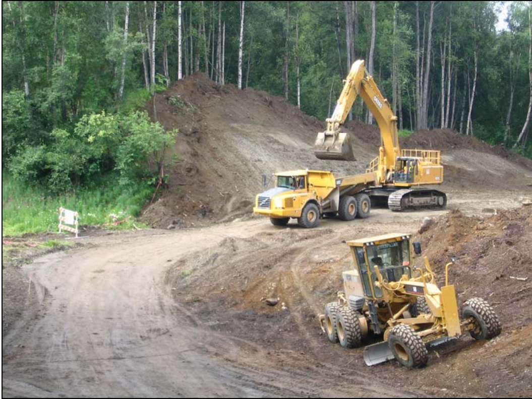
Photo 1. Haul road construction in 2006.
