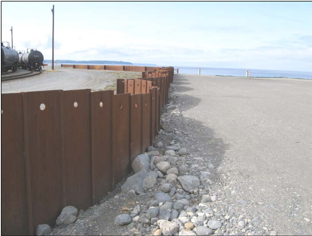
Photo 14. Flint Hills sheet pile wall looking west along the South Backlands.
