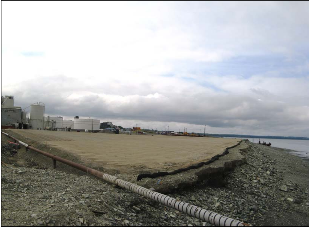
Photo 5. South Backlands in 2008, fill work in progress.
