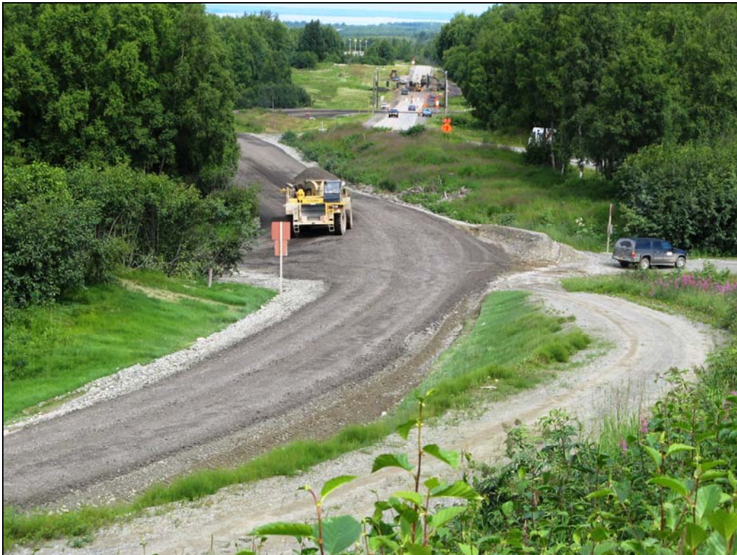
Photo 2. 100-ton haul unit on the completed haul road on Elmendorf Air Force Base.
