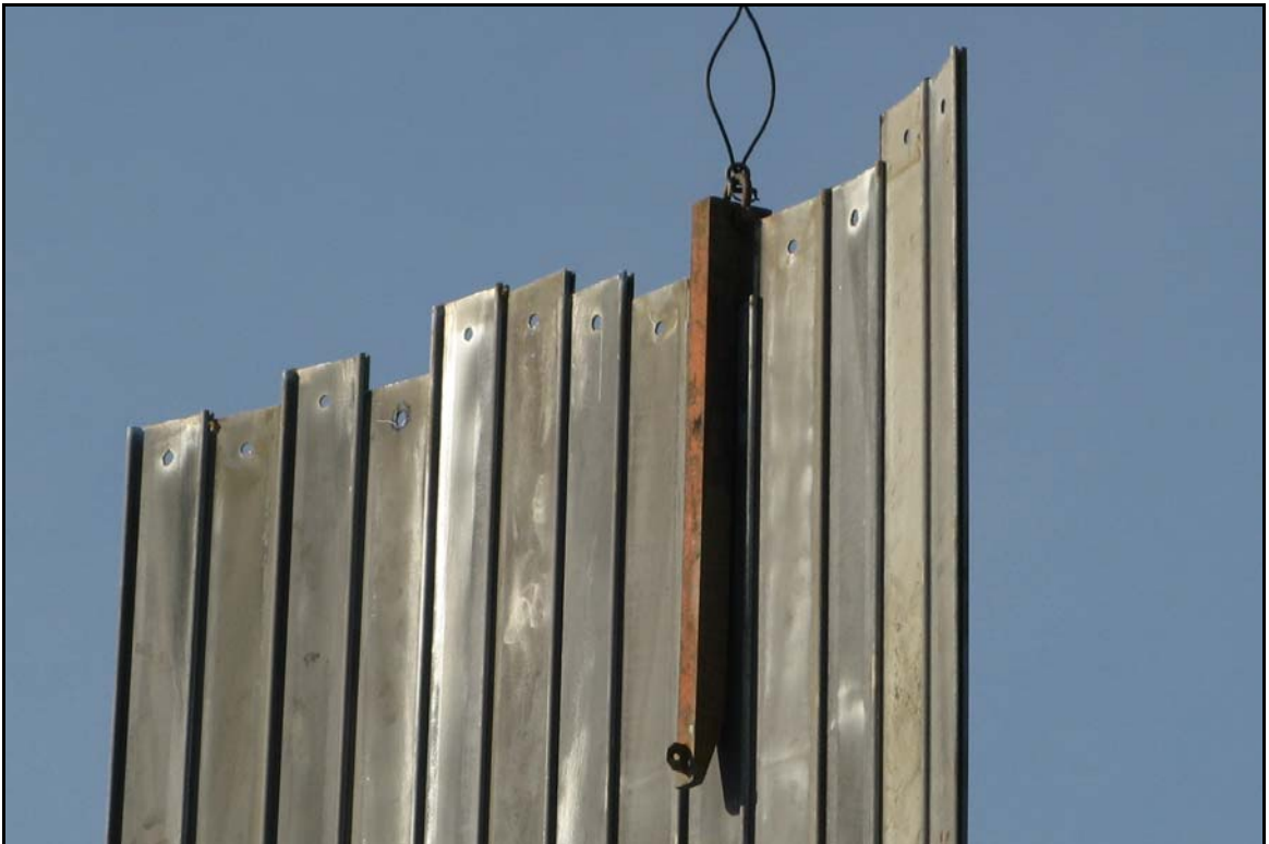
Photo 22. Hairpin weight used to set the sheet pile.
