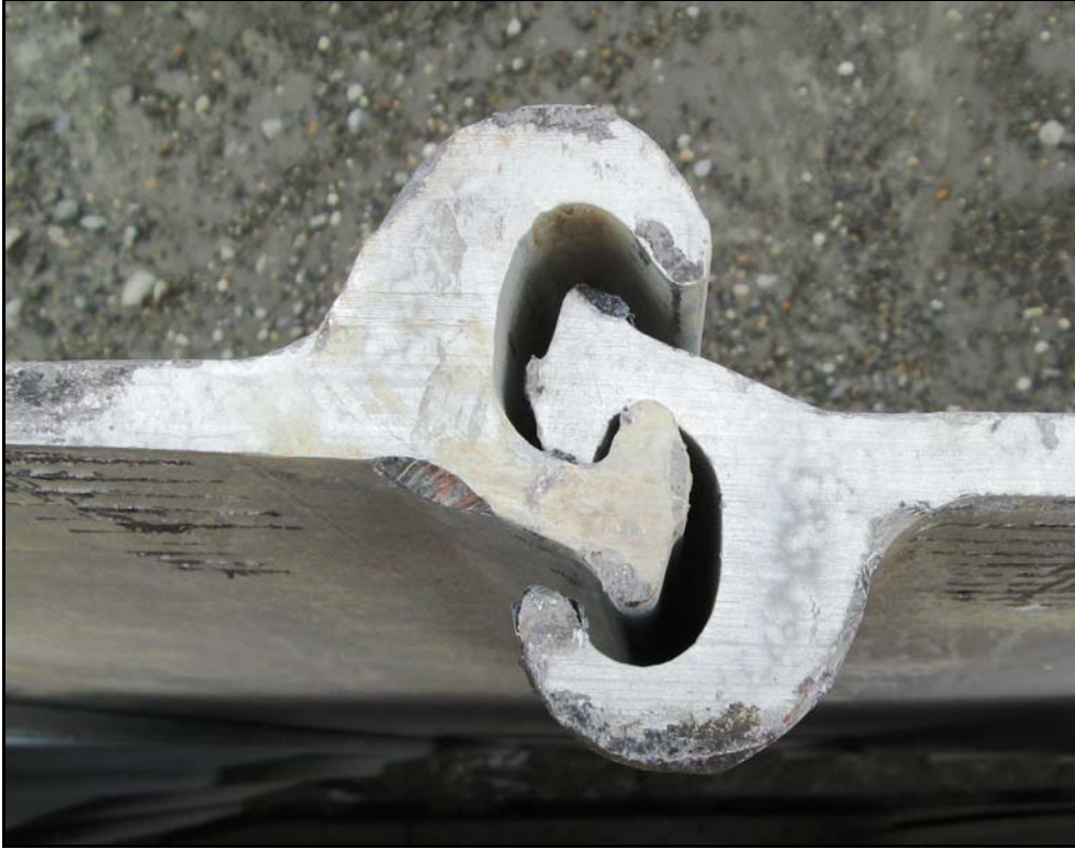
Photo 21. Interlocked sheet pile knuckle joint.
