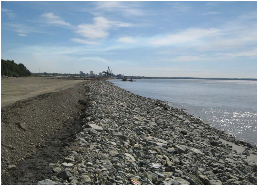
Photo 6. Armor rock north of active docking areas, protects fill from erosion and provides fish habitat. Looking south from northern limit of the Project.
