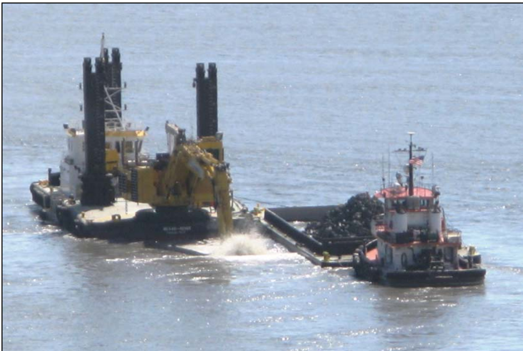
Photo 8. Hydraulic dipper dredge performing construction dredging for the North Extension.
