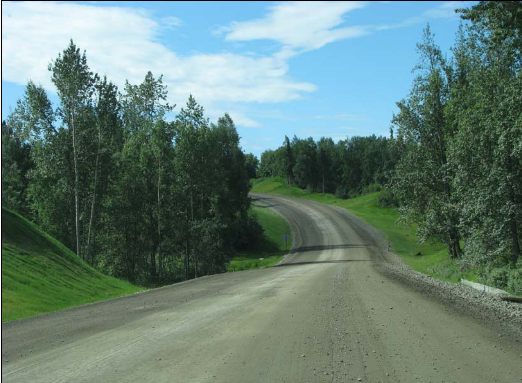
Photo 3. Completed haul road on Elmendorf Air Force Base.
