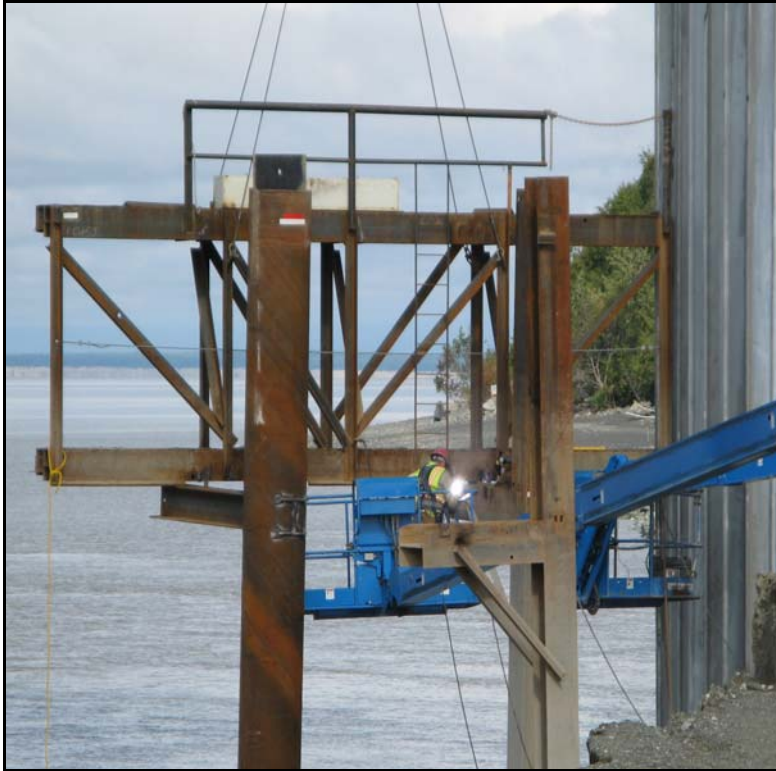
Photo 15. Temporary pile and template.
