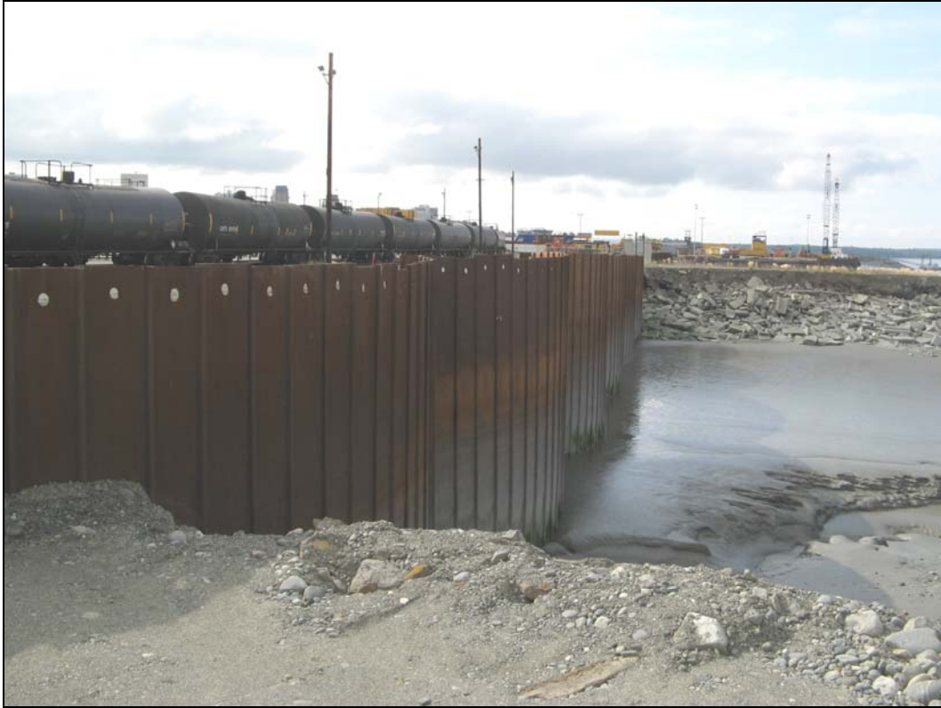
Photo 13. Flint Hills sheet pile wall looking south from the South Backlands.
