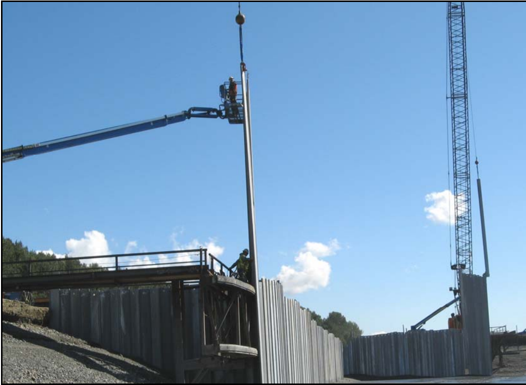
Photo 18. Placing the sheet pile.
