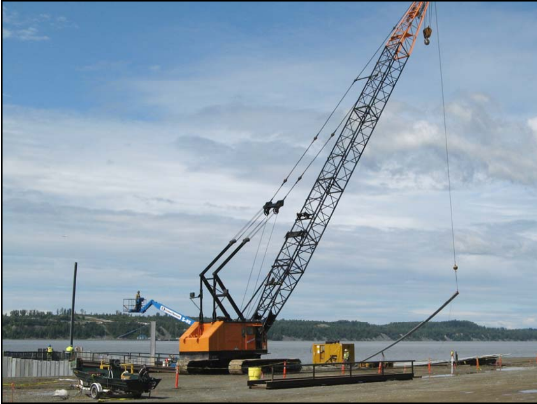
Photo 17. Crane picking up sheet pile.
