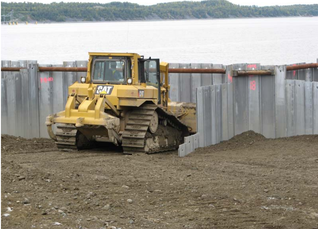
Photo 10. Fill material being placed.
