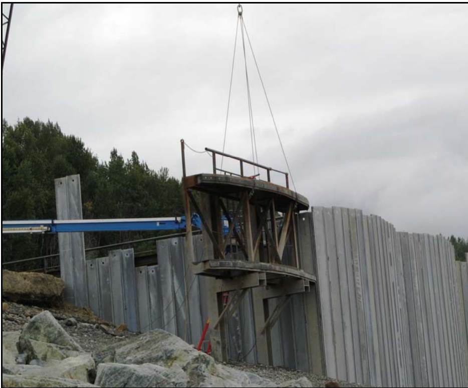
Photo 28. Template and temporary piles are moved to begin the next cell.
