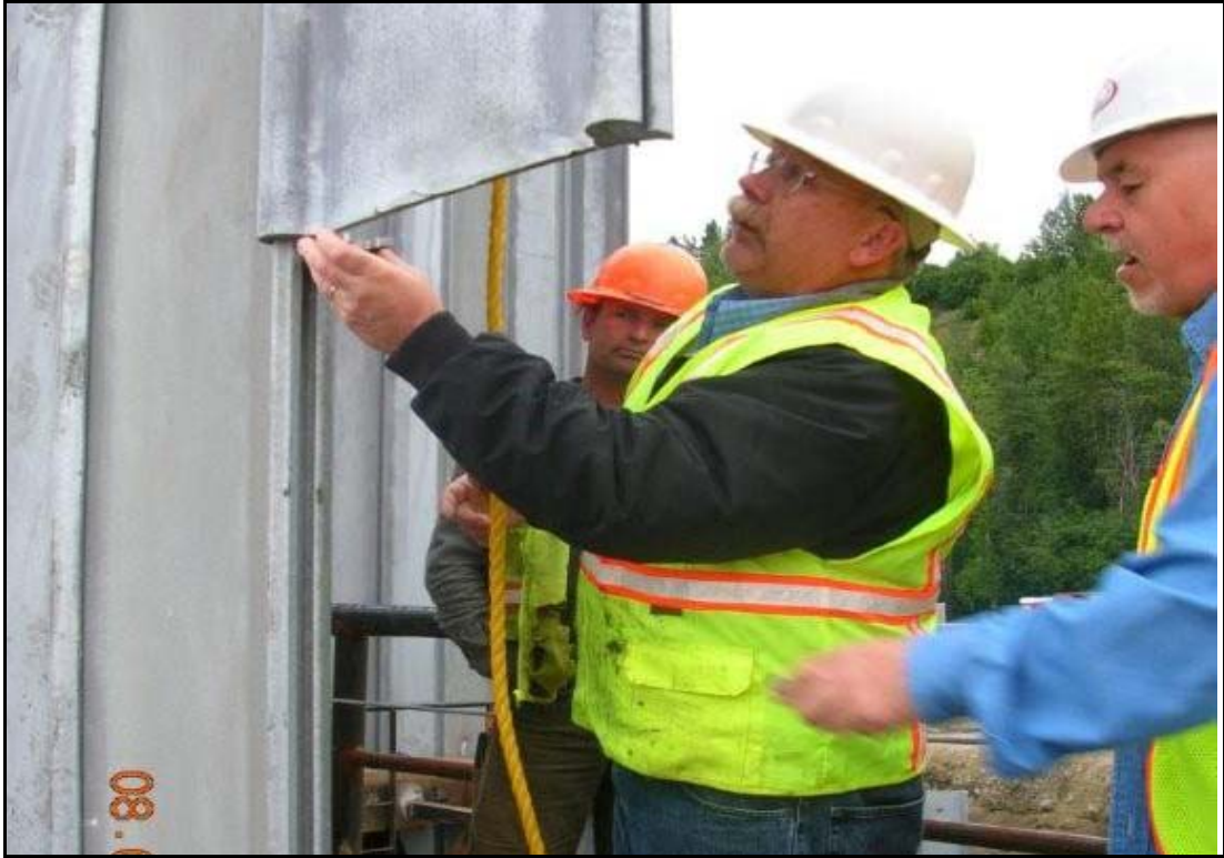
Photo 19. Close up of sheet pile being threaded.
