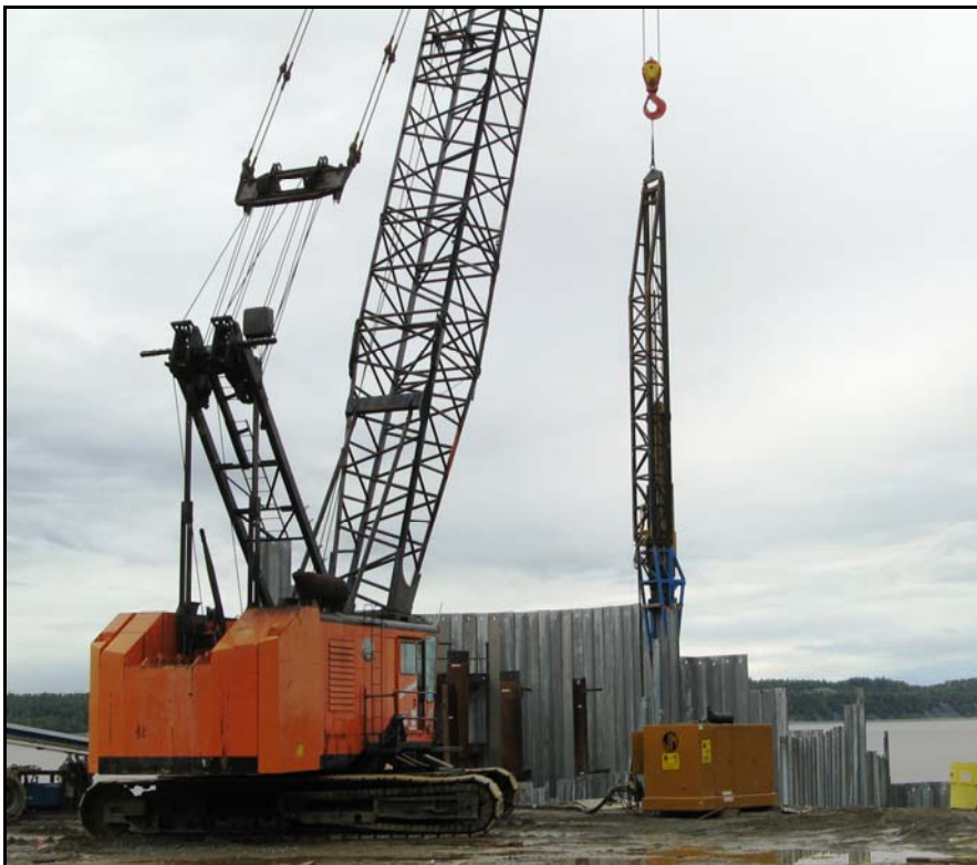
Photo 26. Impact hammer driving the sheet pile.
