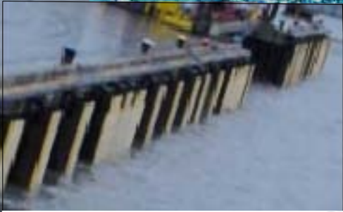
Typical view: Face of existing dock.
