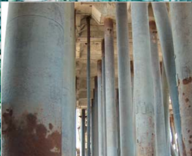
Typical view: Underside of existing steel pile supported concrete deck.
