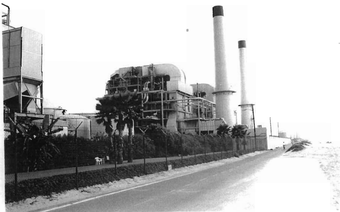
Photograph 3: View of onshore structures of the El Segundo Generating Station.
