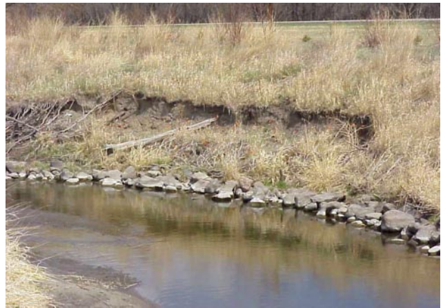
May 2000: High-water events beginning in 1996 scoured out a curve on the riverbank because the radius curvature was too tight for the river to easily navigate.
