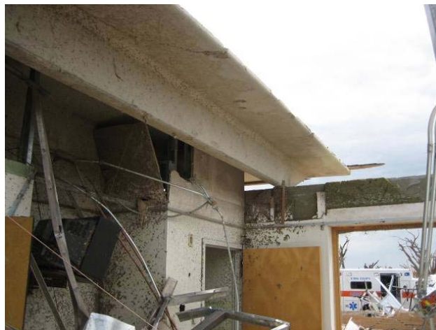
Figure 6: Hospital with Precast Concrete Twin Tees
