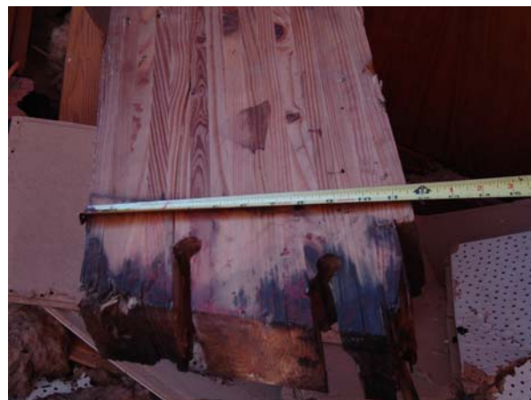
Figure 5: Glulam Beam from Church
