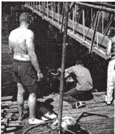
Diver preparing for inspection of Manchester's saltwater pipelines.
